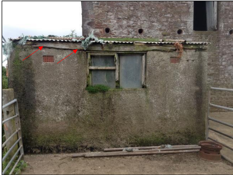
Photo 15: Storeroom attached to the eastern elevation of Building 3. Low potential for supporting roosting bats. Gaps within the wooden barge boarding/lintel may provide a potential roost feature for an opportunistic roost for one or two individuals.
