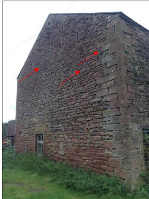
Photo 18: Western elevation of Building 3. Numerous gaps within the stonework across the whole elevation which provide potential access points to roost locations within the stonework (several are indicated with red arrows).
