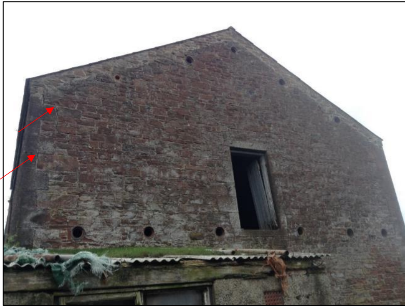
Photo 14: Eastern elevation of Building 3. The stonework is largely well-pointed. However, there are a few gaps surrounding the quoins (as shown by red arrow).
