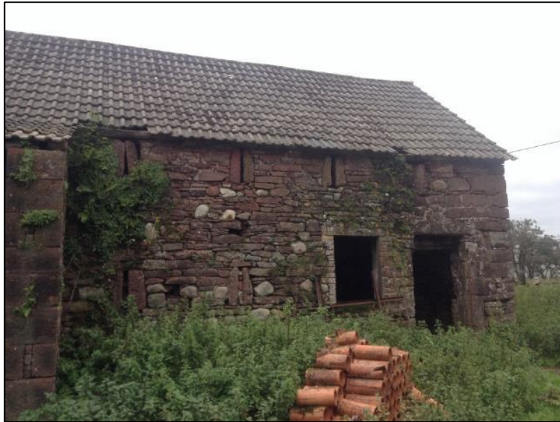
Photo 9: Southern elevation of Building 2. Numerous gaps in the stonework across the whole elevation. Air vents and doorway provide access to internal areas.
