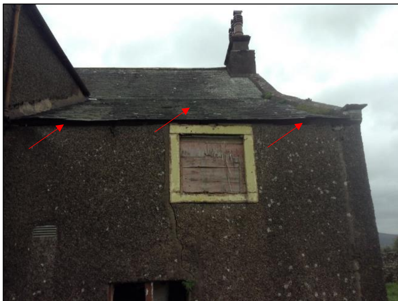
Photo 2: Western elevation of Building 1. Suitable gaps were noted in the exposed stonework at the soffit and under roof slates.
