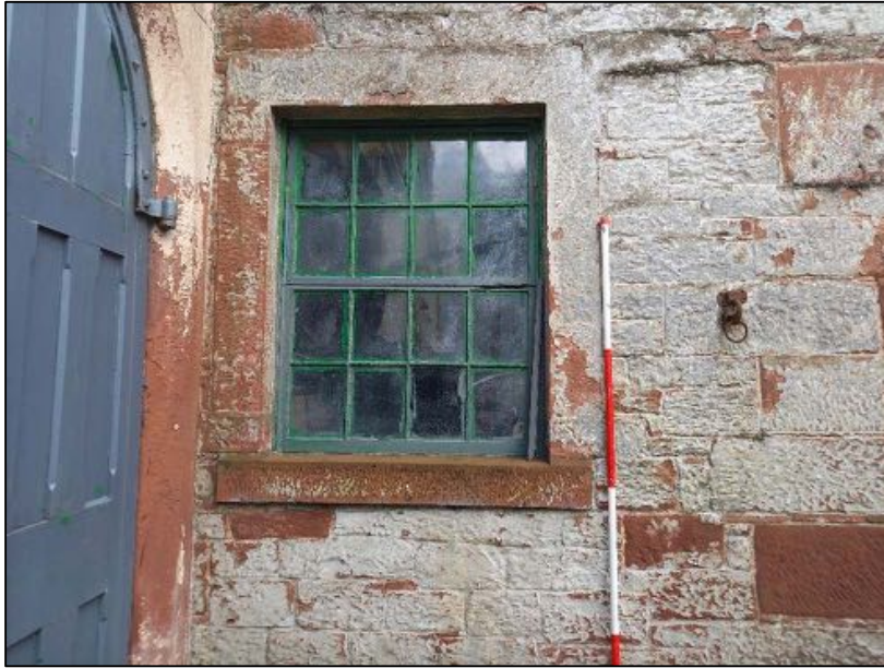
Plate 13: South end of the east elevation of the barn showing possible ground floor stable window
