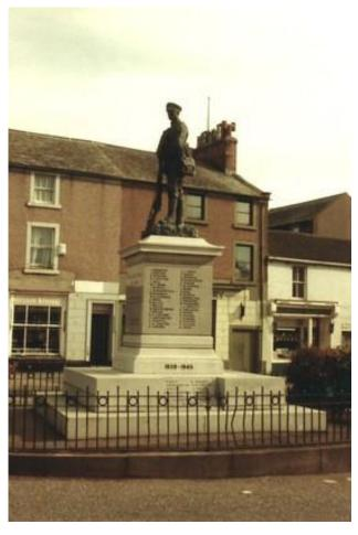
The date of replacement railings is not known, but they appear in a postcard of 1980. A simple design with vertical bars and circles, in mild steel and painted black. The railing panels, fixed to posts at regular intervals, have been curved to fit the curvature of the plinth
