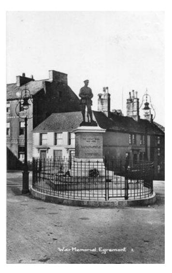
As illustrated in this postcard from C 1930, the original railings were taller than the current railings, approximately 1m high, comprising vertical bars with arrow-type finials, fixed with lead caulk into the kerb stones.
