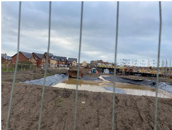
Photograph 20 – Construction site pond
