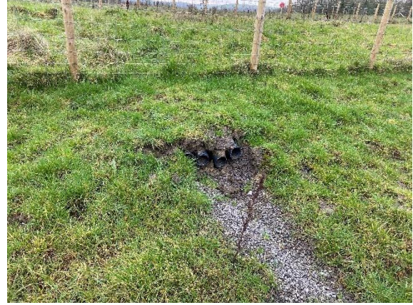
Photograph 19 – Overflow pipes from offsite pond
