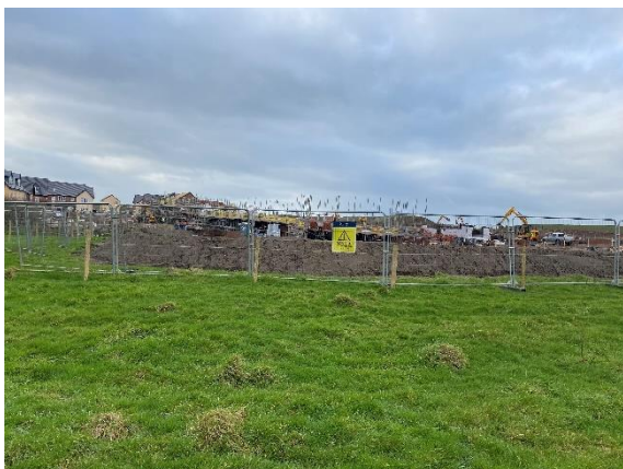
Photograph 16 – Area of construction site encroachment
