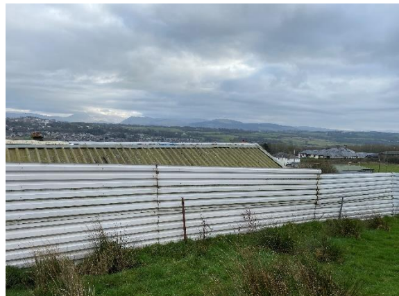
Photograph 11 – Western aspect of land grab fencing
