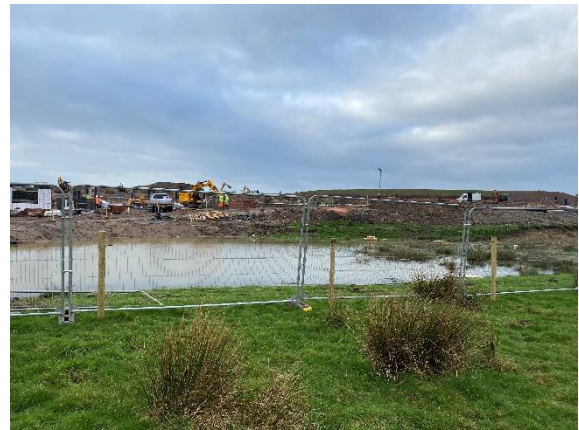
Photograph 21 – Construction site pond
