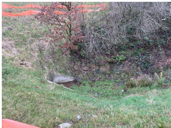
Photograph 5 – Outflow at southern end of ditch
