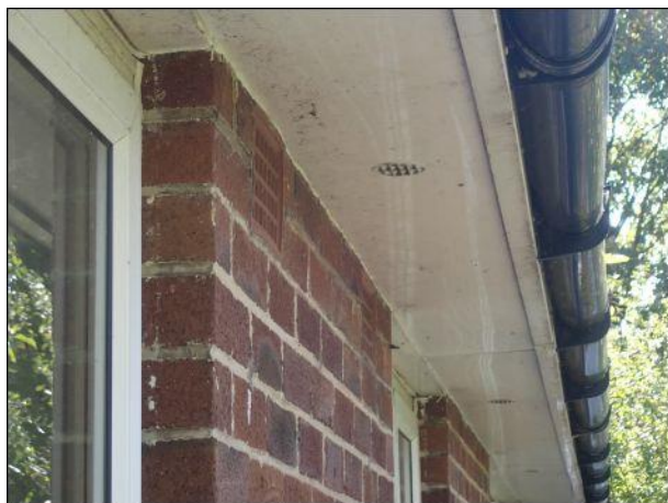
Photo 29: Building 3 well sealed soffits
