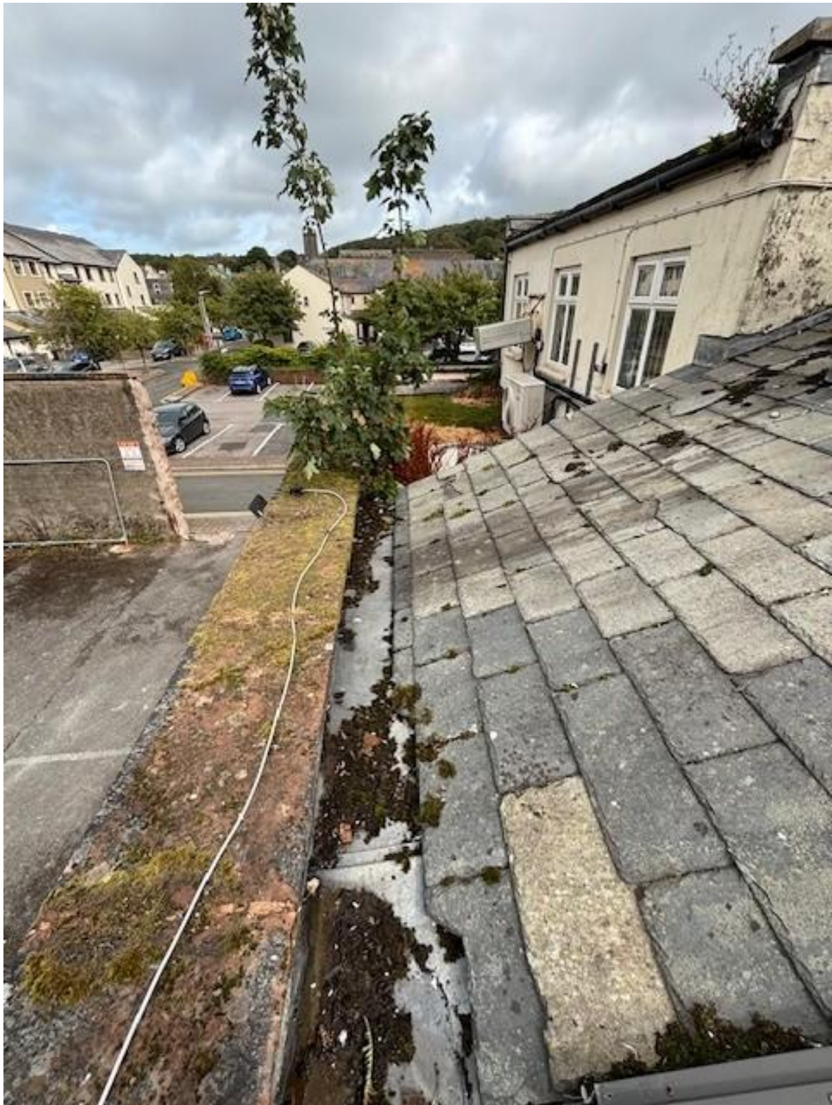
IMAGE 7. VIEW OF PTICED ROOF AND LEAD VALLEY GUTTER FACING FORMER HSBC CAR PARK WITH SINGLE STOREY AND TWO STOREY FLAT ROOFS BEYOND.
