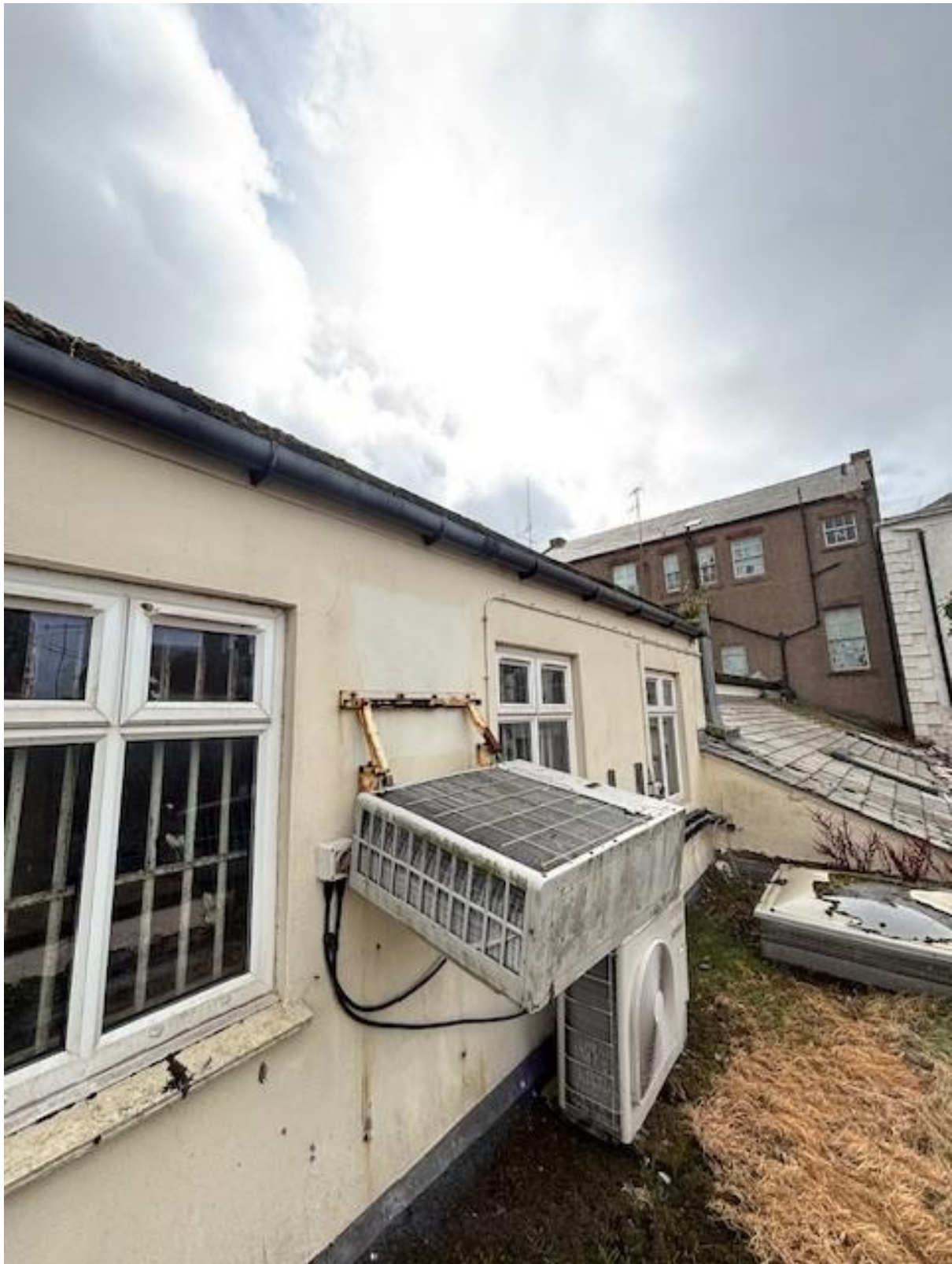
IMAGE 8. VIEW OF TWO STOREY FLAT ROOF SHOWING FASCIA BOARD WITH NO EAVES OVERHANG AND TIGHTLY FINISHED RENDER. THE LEAN-TO PTCHED ROOF BEYOND SHOWS THE UPPER LEAD FLASHING ABUTMENT DETAIL OF THE SLATED LEAN-TO ROOF WITH THE SINGLE STOREY FLAT ROOF.
