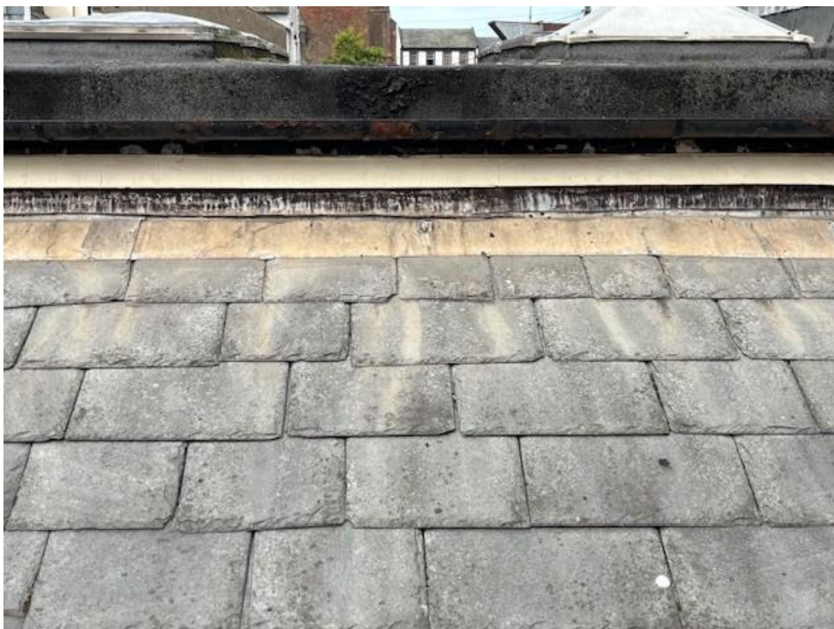
IMAGE 4. VIEW OF PITCHED ROOF SHOWING LEAD FLASHING ABUTMENT AND TIGHTLY FITTING SLATE.
