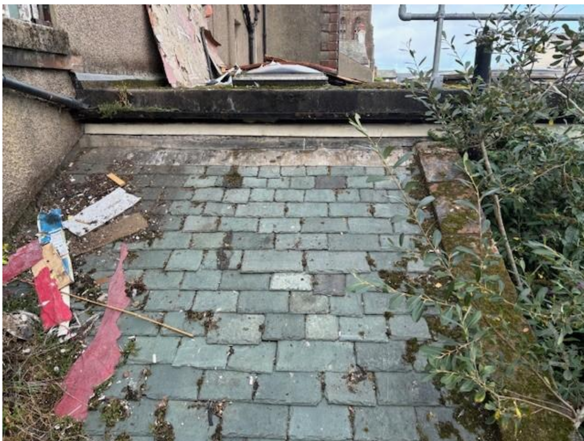
IMAGE 3. VIEW OF PITCHED ROOF SHOWING LEAD FLASHING ABUTMENT, PARAPET WALL AND TIGHTLY FITTING SLATE.
