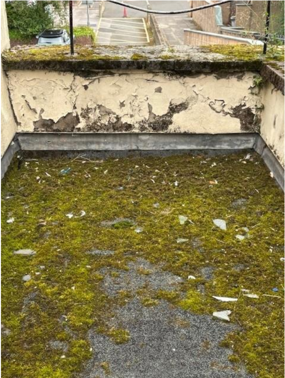
IMAGE 5. VIEW OF CONTAINED FLAT ROOF FACING SCHOOLHOUSE LANE WITH PARAPET WALLS ON ALL SIDES AND LEAD FLASHING ABUTMENT.
