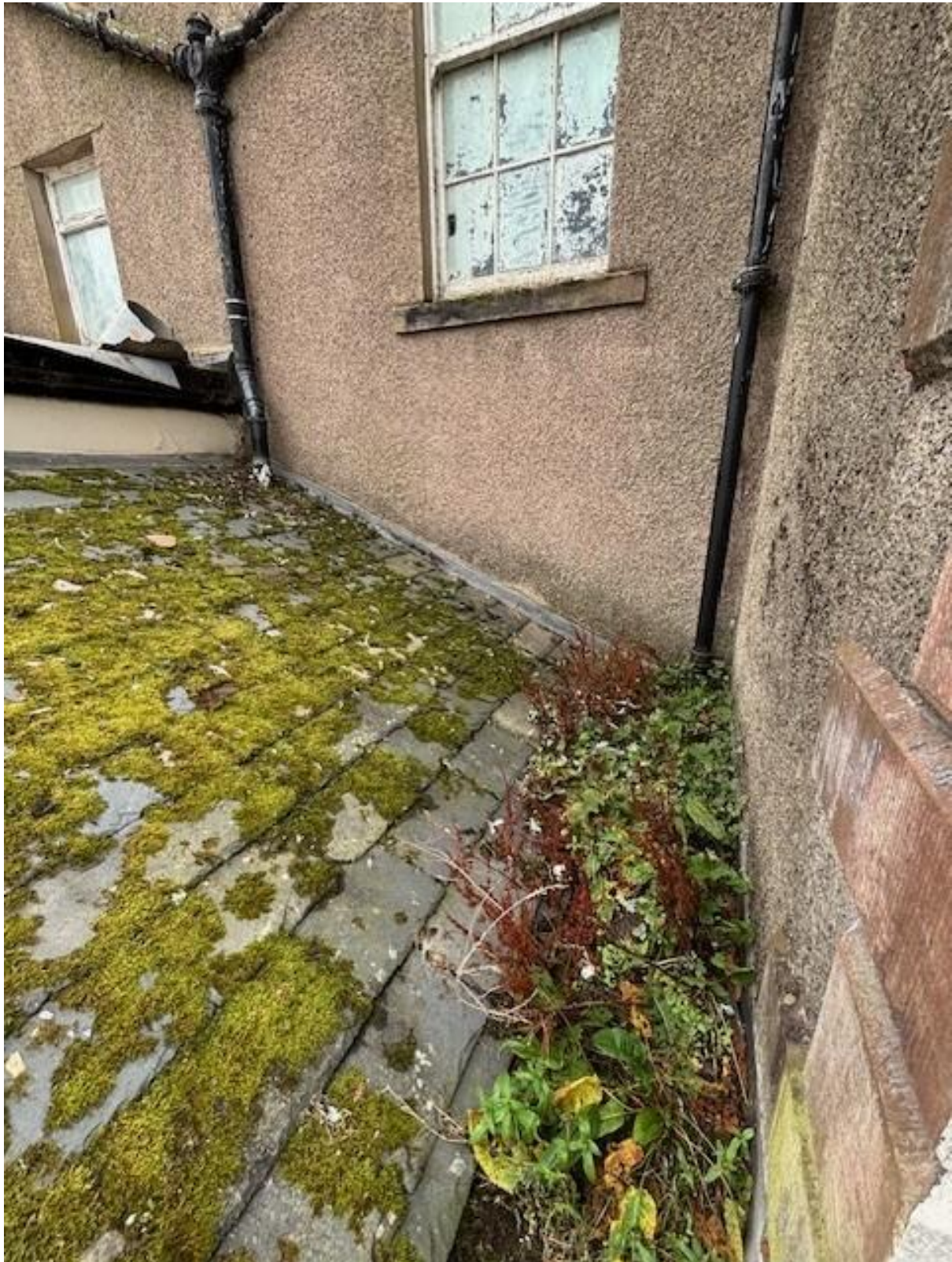
IMAGE 9. LEAN-TO PITCHED SLATE ROOF ABUTMENT WITH MAIN 3-STOREY REAR WALL SHOWING UPPER LEAD FLASHING ABUTMENT, LEAD VALLEY GUTTER AND TIGHTLY FITTING SLATE.
