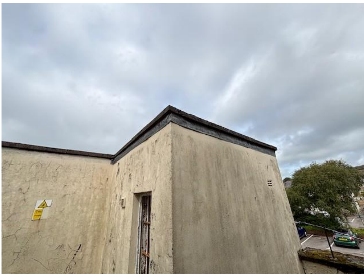
IMAGE 6. VIEW OF TWO STOREY FLAT ROOF SHOWING FASCIA BOARD WITH NO OVERHANG AND TIGHTLY FINISHED RENDER.
