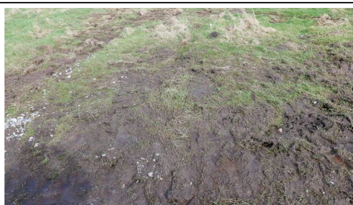
8. Typical ground conditions
