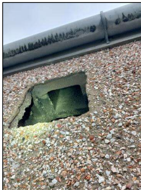
Photograph 2 Hole leading into cavity of breeze block of building reference B.
