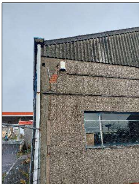
Photograph 3 Missing render, hole and cracks all providing potential for roosting bats.
