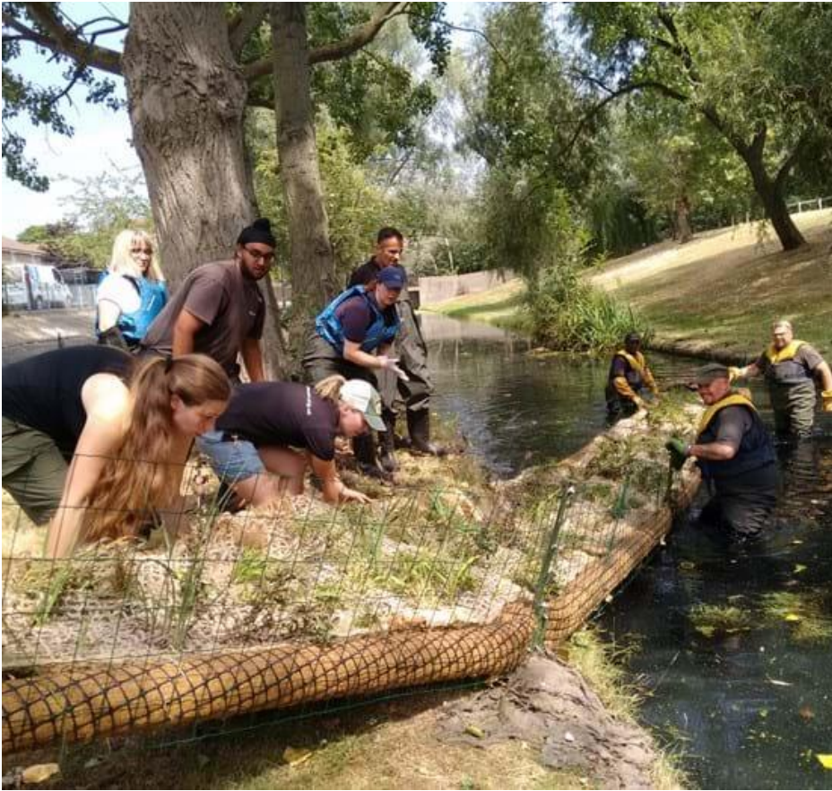
Figure 9.11 Thamesmead volunteer programme building floating reedbeds
