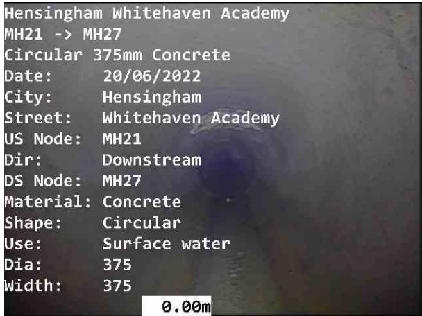
MH21X_a6486355-cf25-403d-a166-47ba39500958_20220622_153706_376.jpg, 00:00:00, 0.00 m Start node, manhole, reference: MH21
