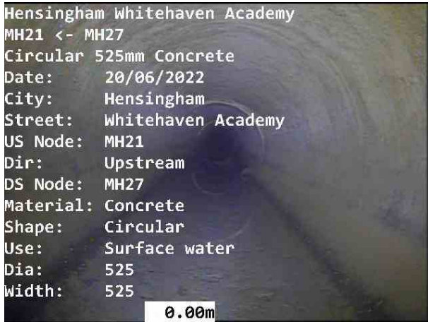
MH21X_ce390d49-0f25-447a-8f10-d813b35b3e71_20220622_153449_770.jpg, 00:00:00, 0.00 m Start node, manhole, reference: MH27
