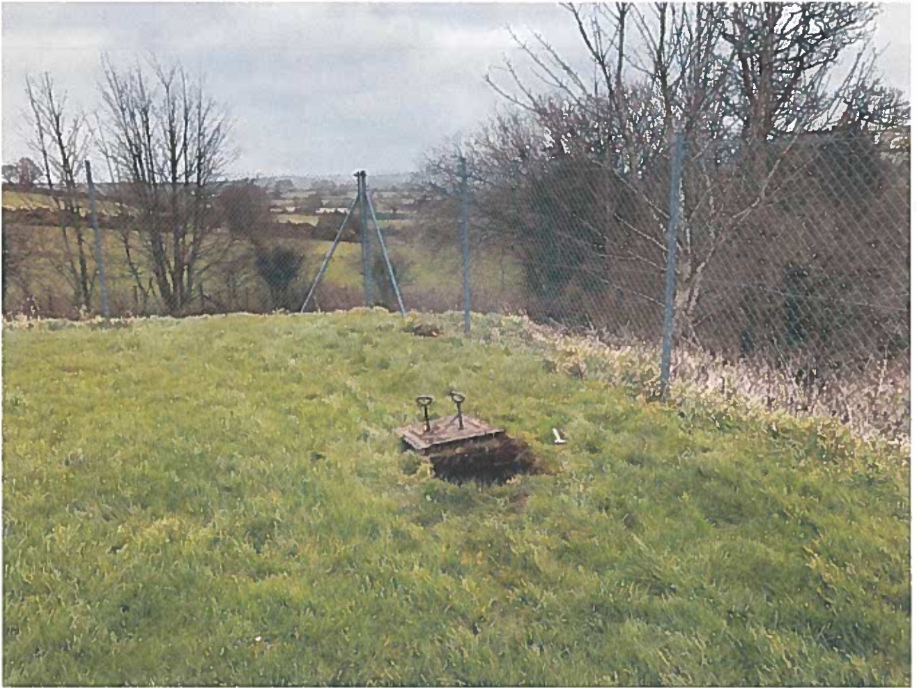
Manhole towards eastern boundary
