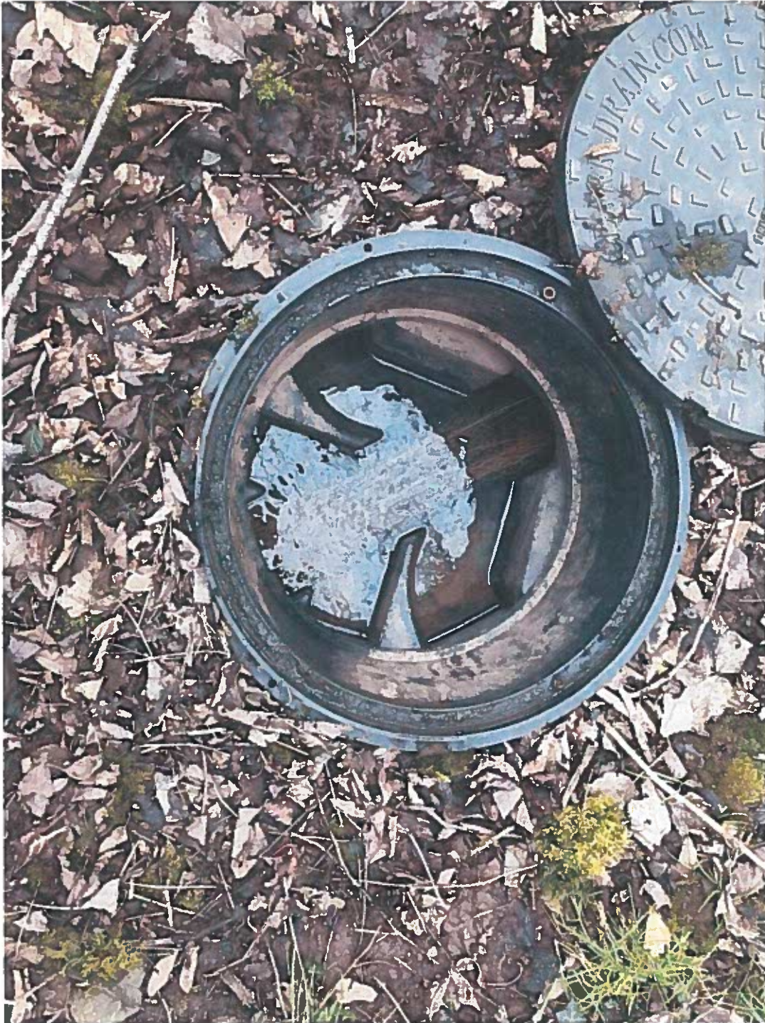
Final Outfall from site
