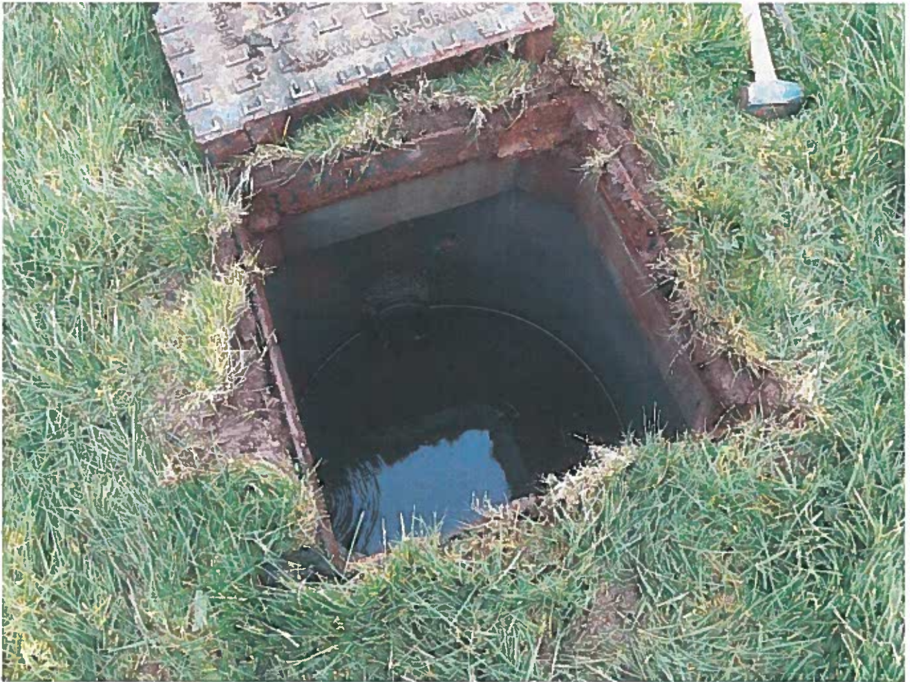
Manhole Adjacent to eastern boundary
