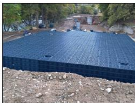
Housing Estate, Aberdeenshire (UK)
