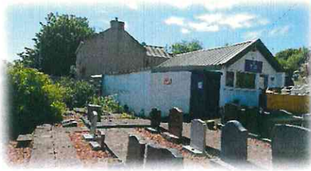
Plate 1: External view of Garage.
