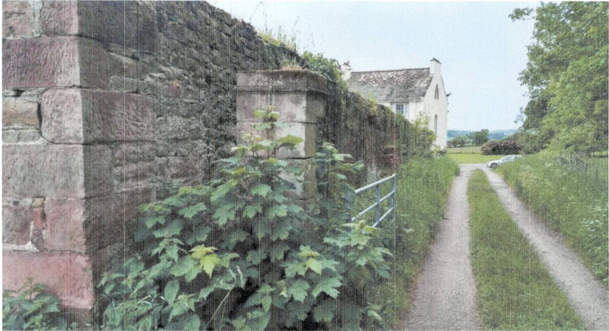
It would appear reasonable to view this pair of gate piers as falling within the curtilage of the listed house. These sycamore saplings need removing to avoid destabilising the gate pier.
