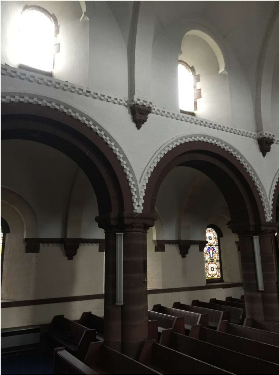
Figure 3: Internal detailing to be retained.
