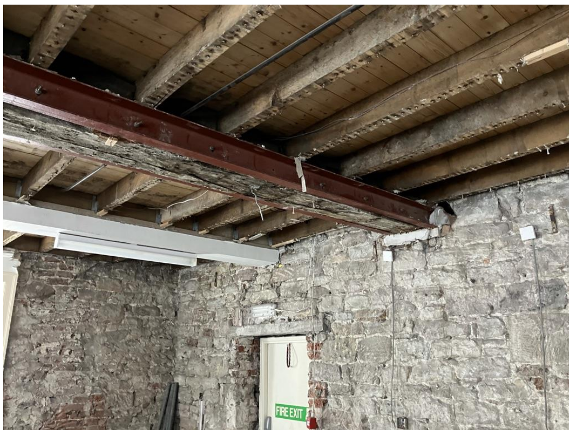
Strengthening works to existing timber beams
