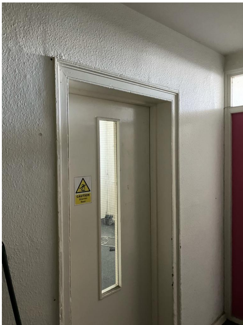
View of internal doorway into the front of Apartment 2
