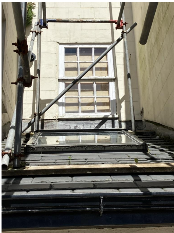
Modern timber window replacement – softwood mock sash window with lower hung casement window, lean to slate roof below
