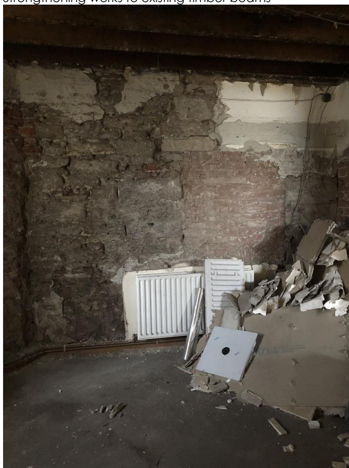
Gypsum based modern plaster and plasterboard removed from external walls.
