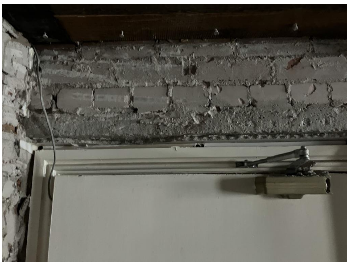
Internal view of rear doorway into Apartment 2
