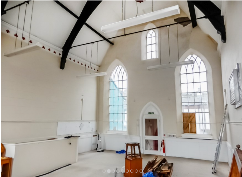
Above photograph showing decorative woodwork and ceiling trusses which will be retained.
