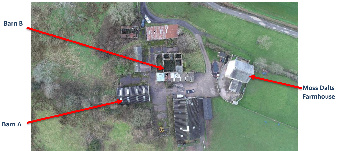
Fig 2 –Aerial image of site
