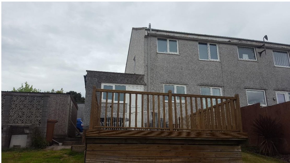
Photo 2 – Photo of Rear (West Elevation)
