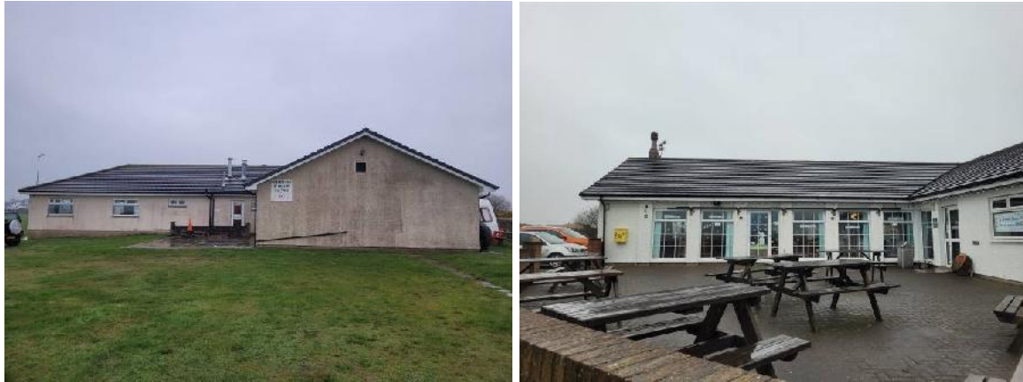
(Fig.08-17 – Images of the existing building from various camera angles)
