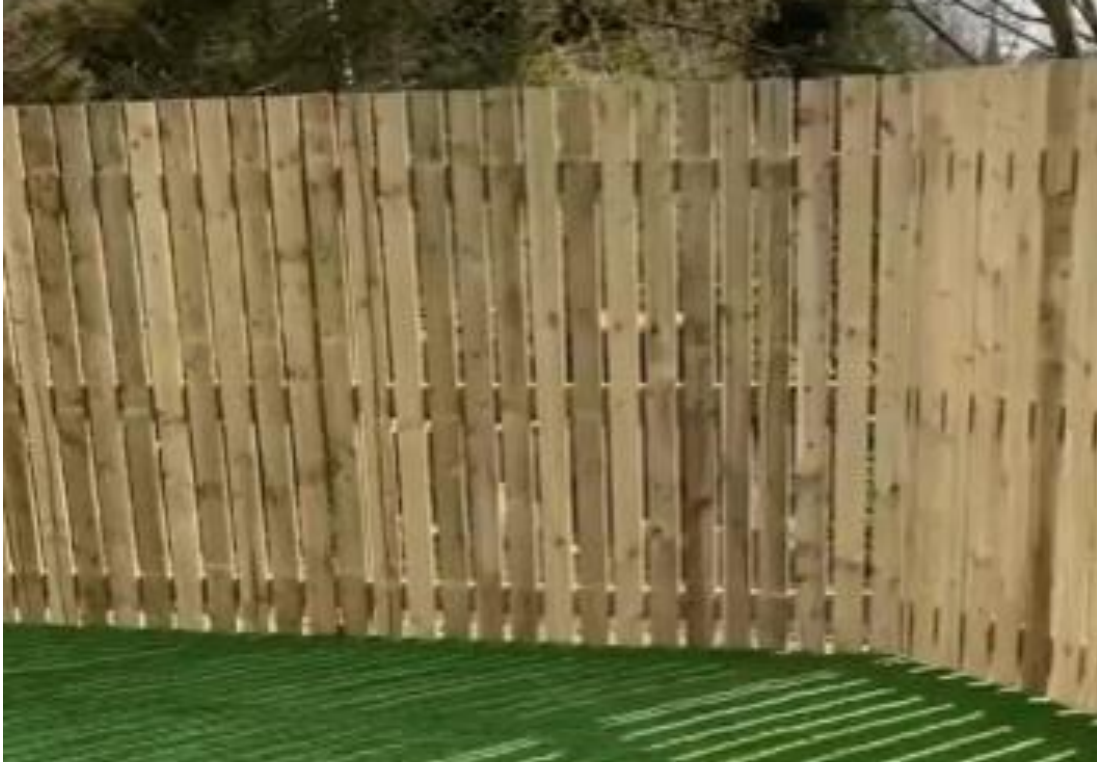
1.8m timber hit and miss fence to rear side boundaries
