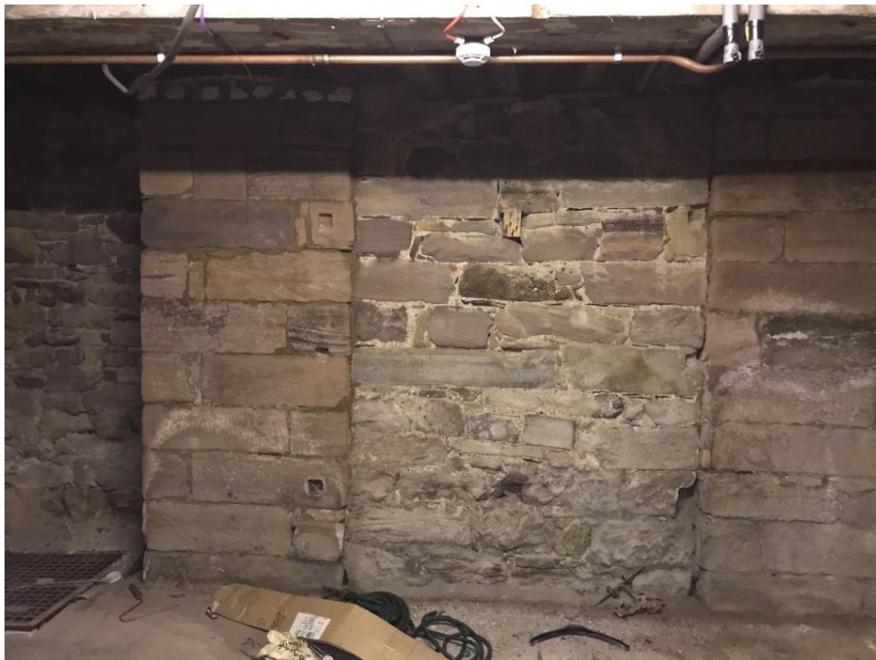
Basement area under the main building
