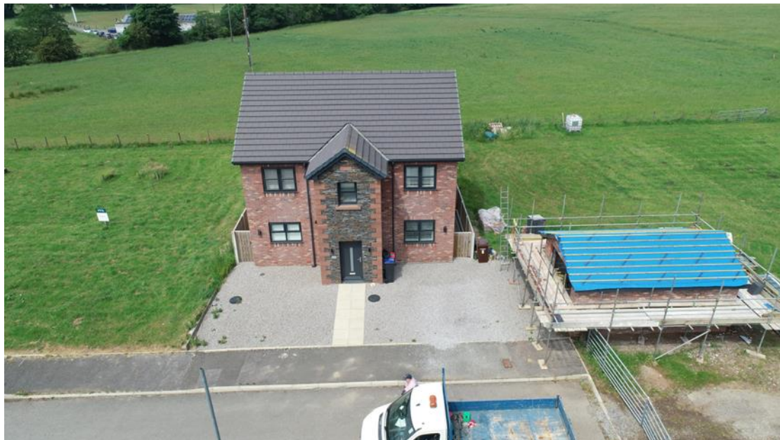
Photo 8 – Aerial Photo of Plot 6 Church Crescent
