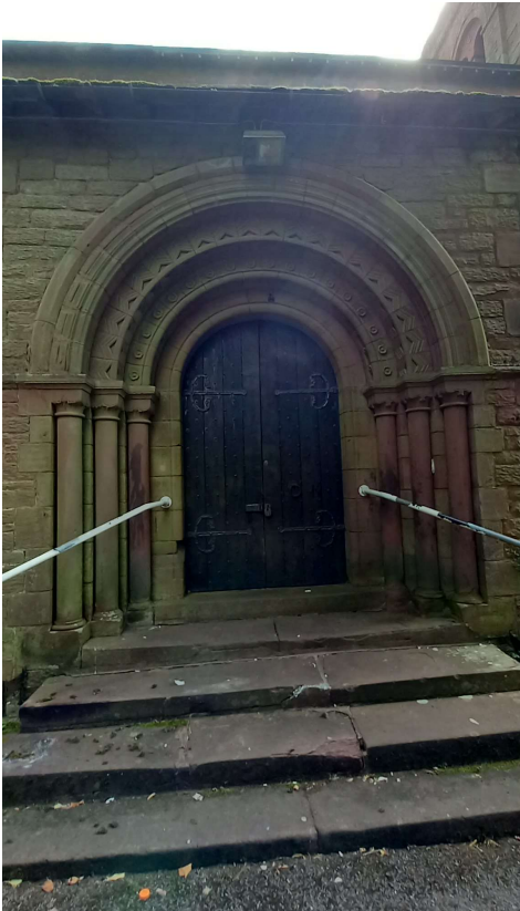
Fig.6 - Existing Stepped Entrance.
