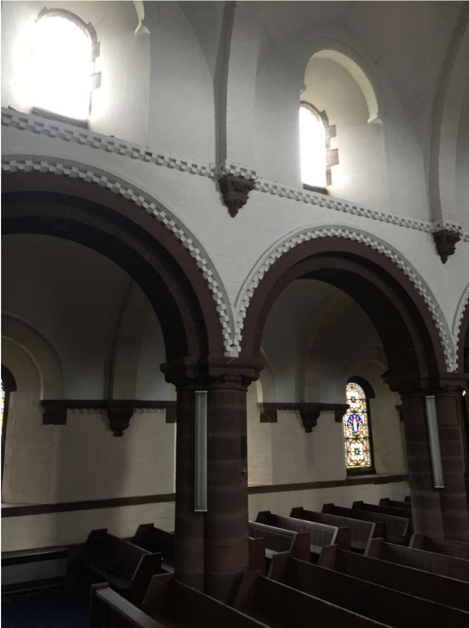
Figure 3: Internal detailing to be retained.
