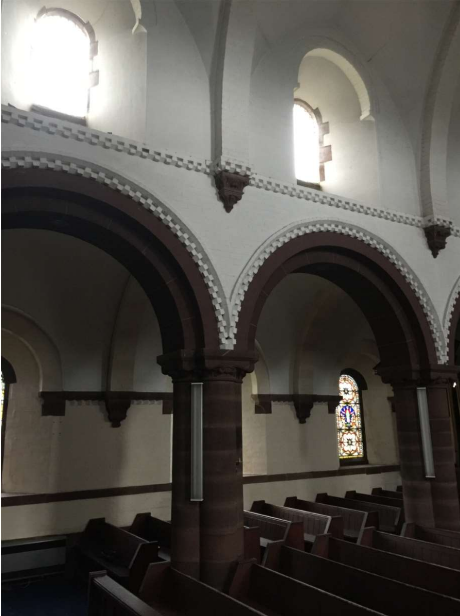
Figure 3: Internal detailing to be retained.
