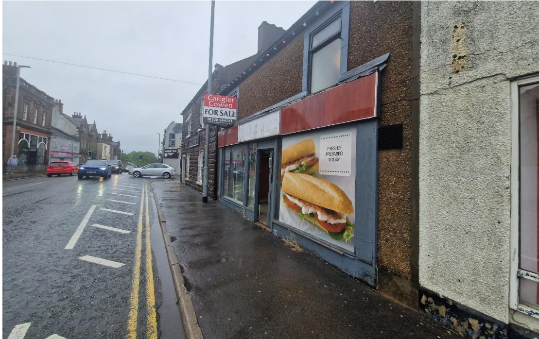
Photo 9 – Existing Ground Floor Windows & Door – Grey Timber & Aluminium
