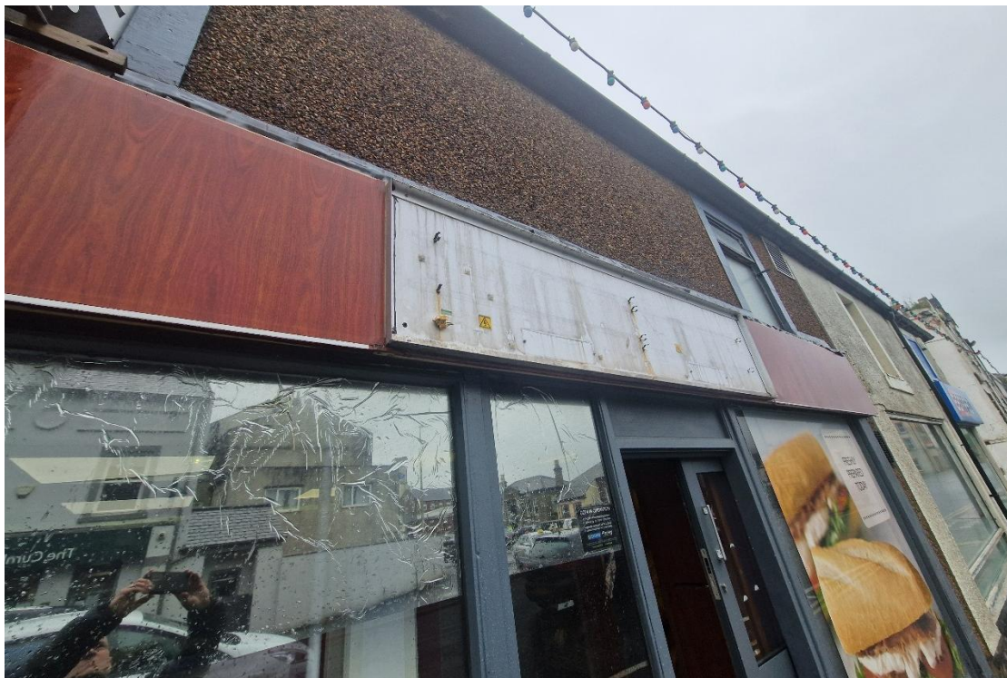
Photo 4 – Existing Upper & Ground Floor Window – Grey Timber & Aluminium
