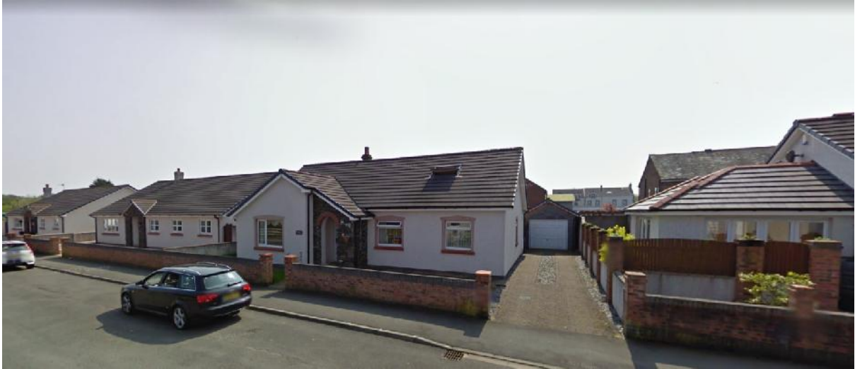
Fig. 15 – Single Storey detached dwellings along Millom Road)
