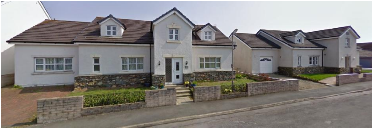
(Fig. 12 – Detached dwellings fronting King Street)
