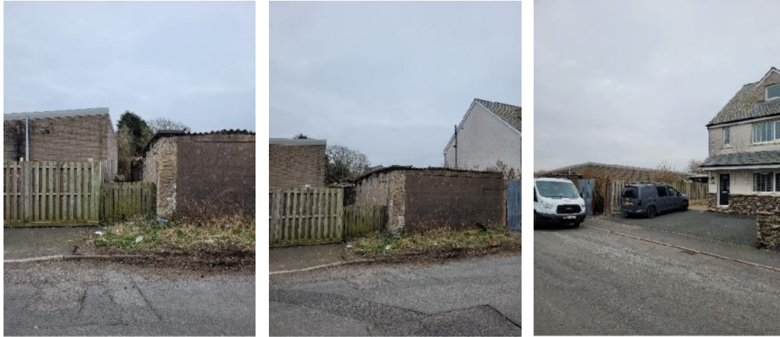
(Figs.08-10 – Existing Images of the Application Site along King Street)
