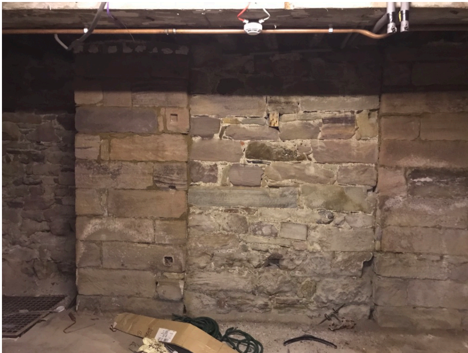
Basement area under the main building
