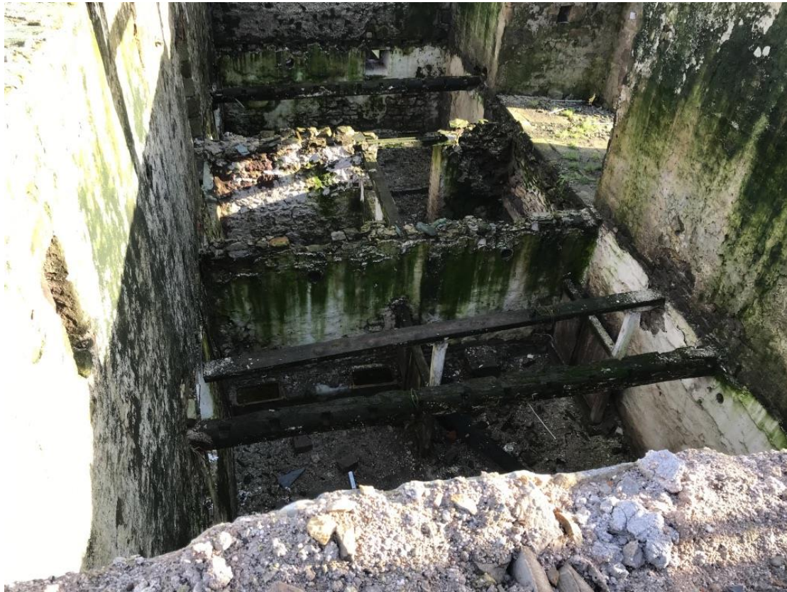
View internally from the West – flanking wall to left hand side requires re-building
