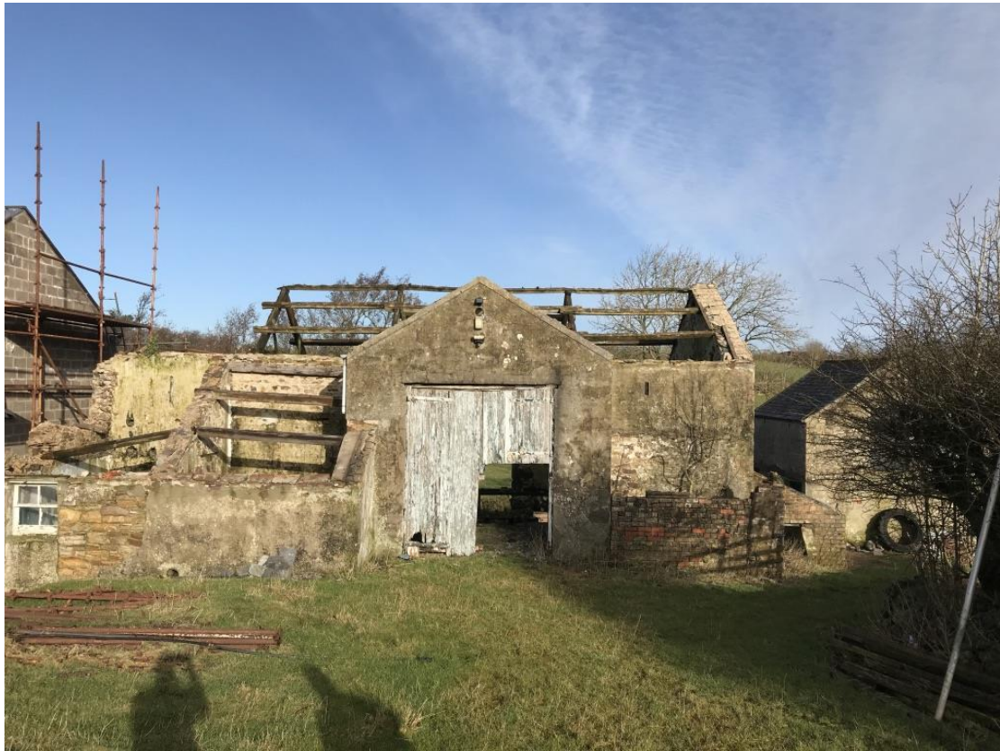
Rear elevation with roof stripped to reduce weight on existing walls
