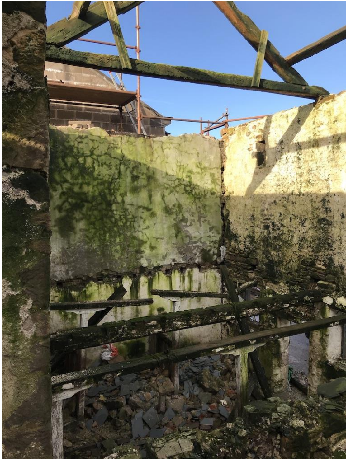
Internal view of the floor with rotten floors removed
