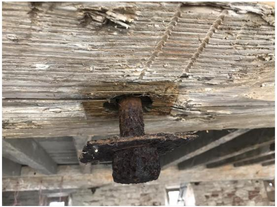
Steel bars forming roof truss have separated from lower chord as whole truss has rotated as decay has set in, separation 35mm
