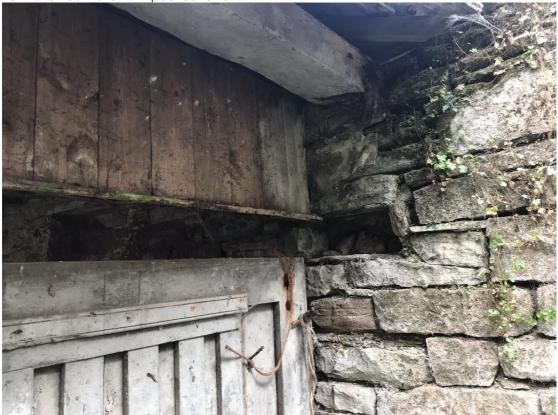
Pockets in stonework iodentifiying locations of timber lintels long since rotted away, exposed rafter feet on roof shown above.
