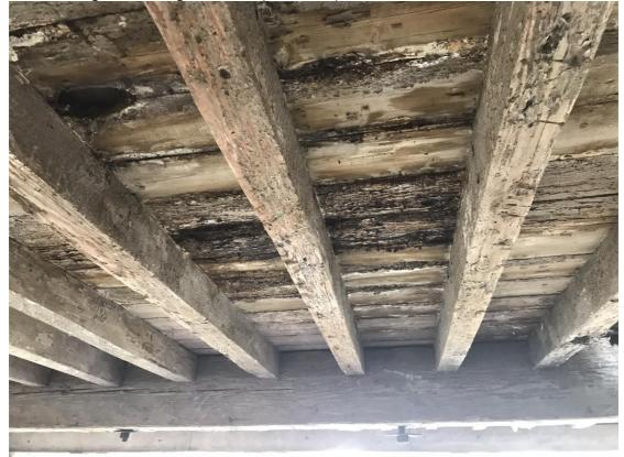
Water damage to floor boards – now soft with wet rot
