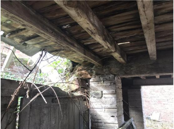
Floor overhanging at first floor level, with lower course of slates showing as valley and elad work has disappeared / rotted away.
