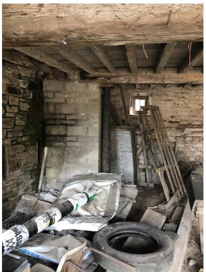
Rear left hand masonry column, timber beam decayed and rotted at valley junction
