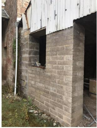
Left hand side opening shortened in width circa 2m to support bearing of new steel beam
