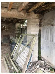
Modern internal block piers supporting decayed end of the timber
