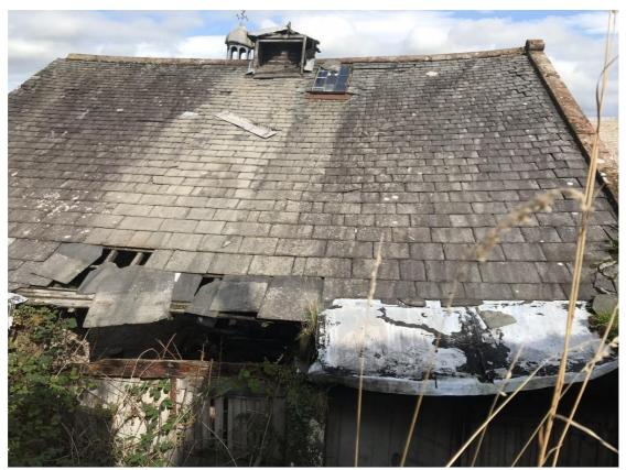
Part of lead valley in situ, rotation of truss evidences with ridge dropping sway from rear wall, ventilation cowl shown in poor condition.
