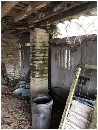
Side gable of barn, lead valley and horizontal timber beams now rotted and absent on site
