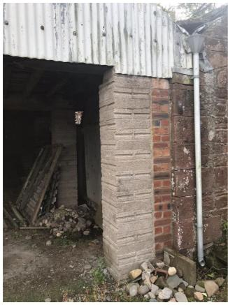
Right hand column of ginnery supported on new masonry columns
