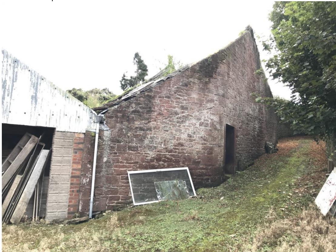
Existing rear barn with roof removed forms new garden area, access lane to walled garden remains
