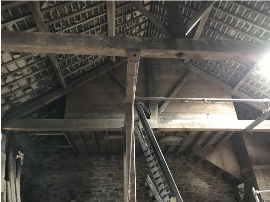
Existing loft are within the trusses forming pigeon loft
