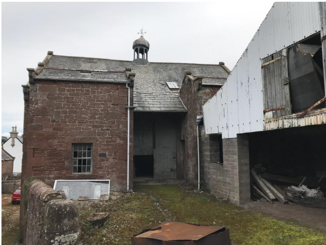
Rear elevation with Georgian windows and modern barn
