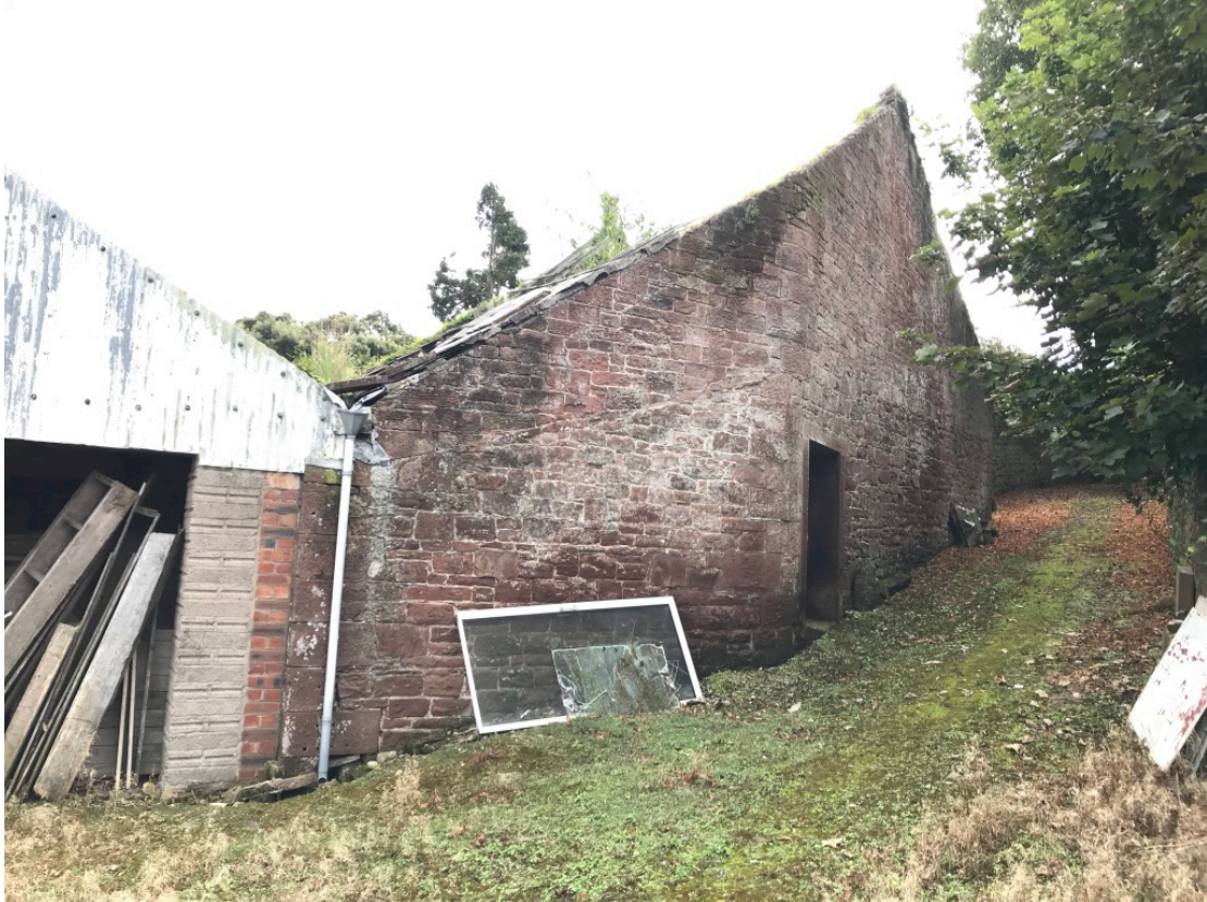
Existing rear barn with roof removed forms new garden area, access lane to walled garden remains
