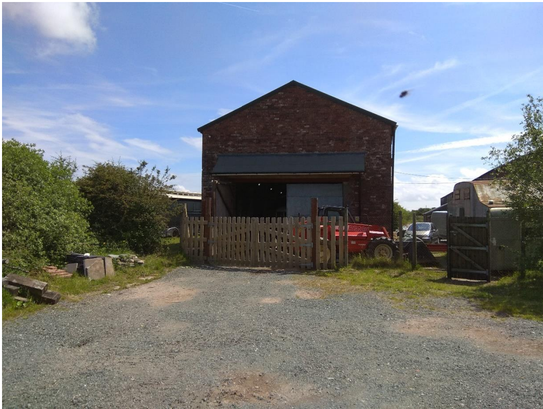
Photo 6 & 7 – Existing West Elevation
