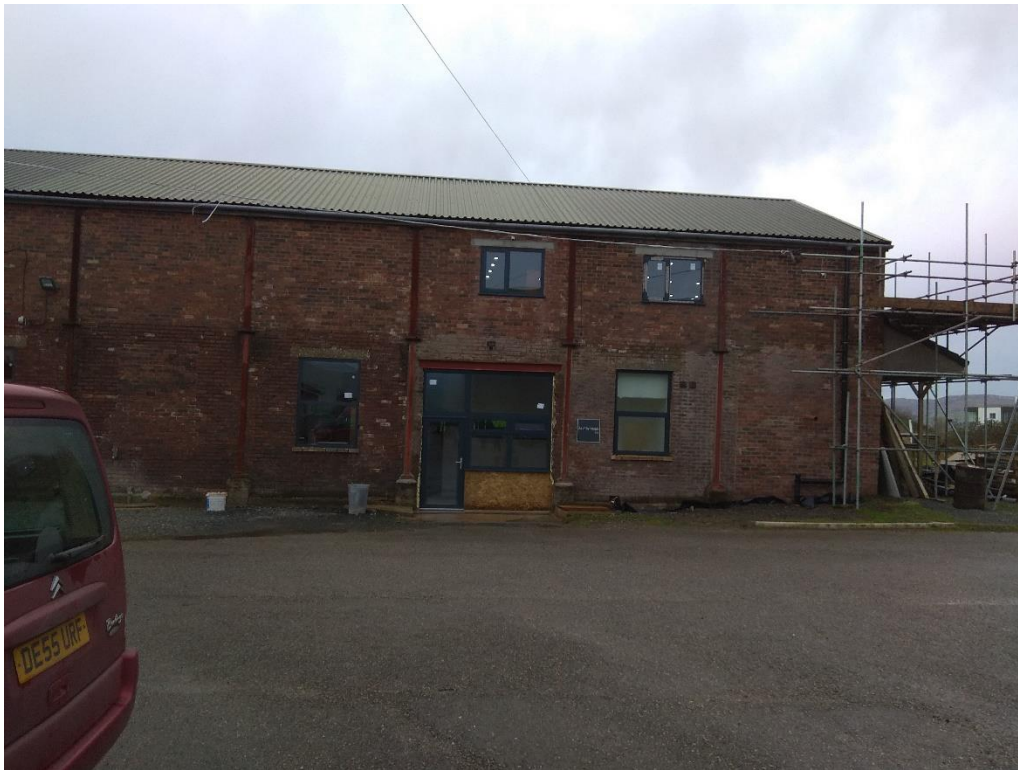
Photo 1 & 2 – Existing South Elevation (Main Entrance)
