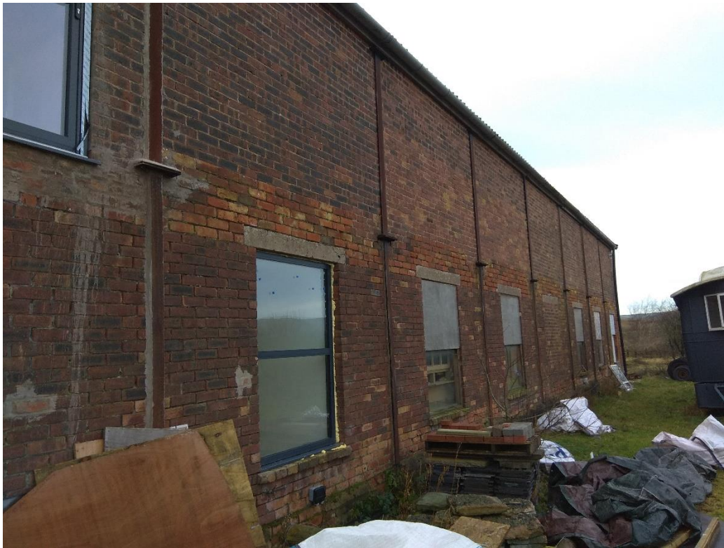
Photo 5 – Existing North Elevation (location of proposed extension)
