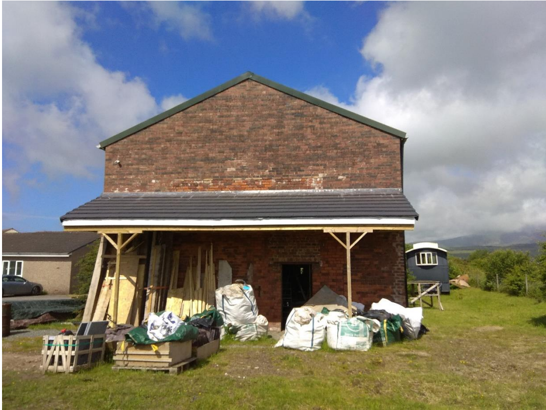
Photo 3 & 4 – Existing East Elevation
