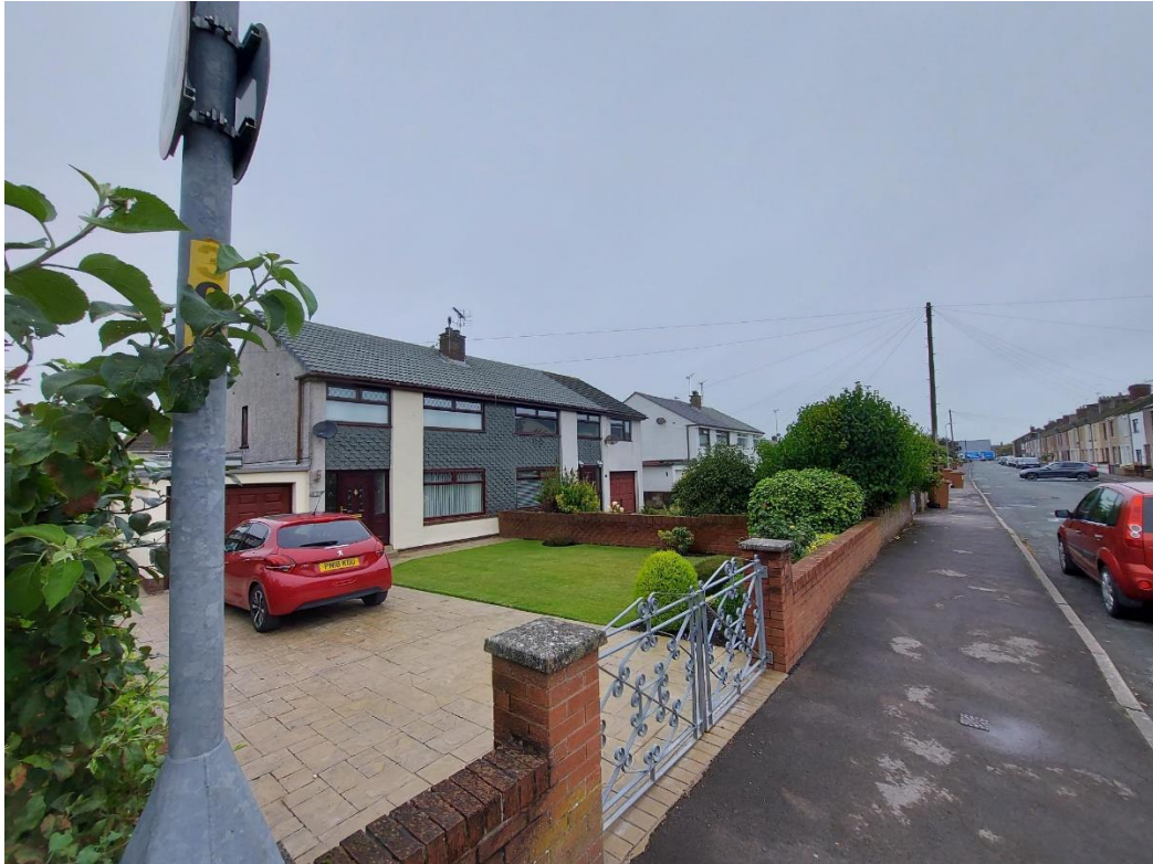
Figure 6 - A house finished in hanging slates, slate grey concrete roof tiles and light render (3 Mainsgate Road, Millom)
