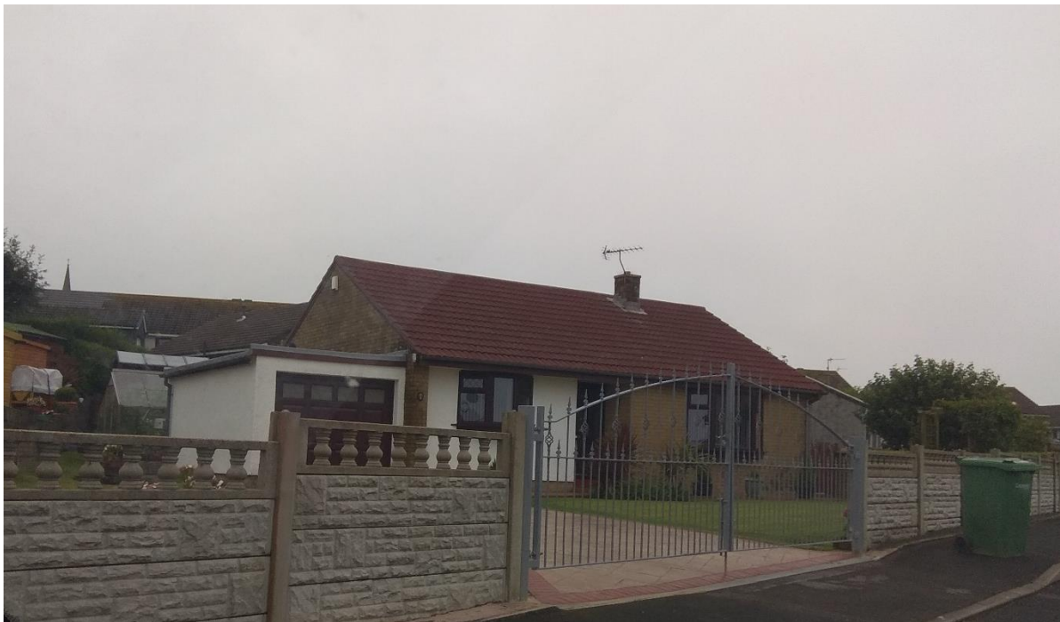
Figure 3 - A bungalow finished in red tiles, yellow brick, and smooth white render (1 Thirlmere Close, Millom)
