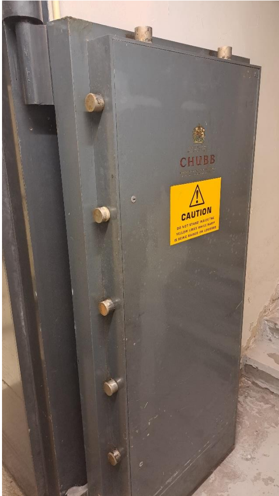
Figure 3 Strong door within basement corridor
