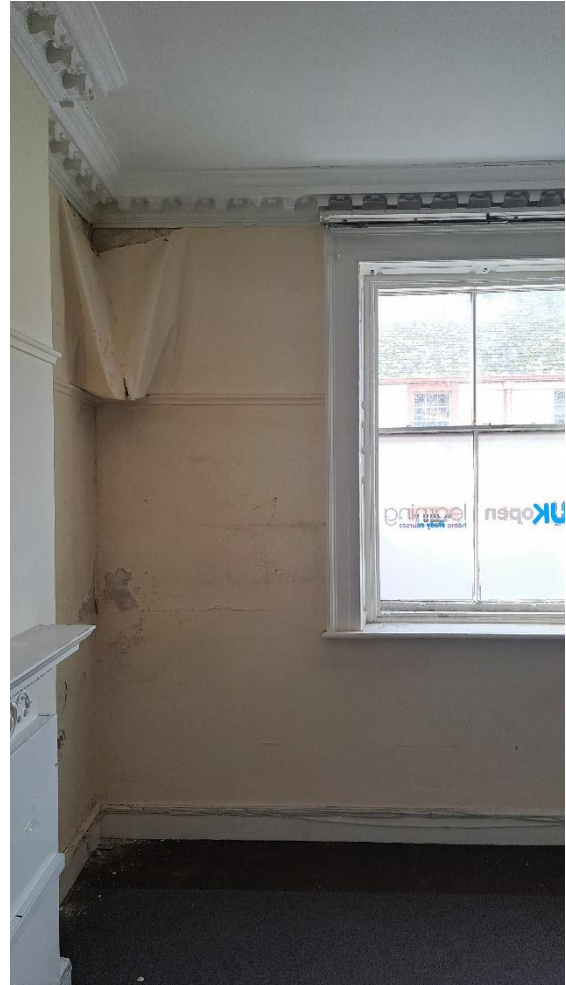
Figure 8 Moulded cornicing (much overpainted)
