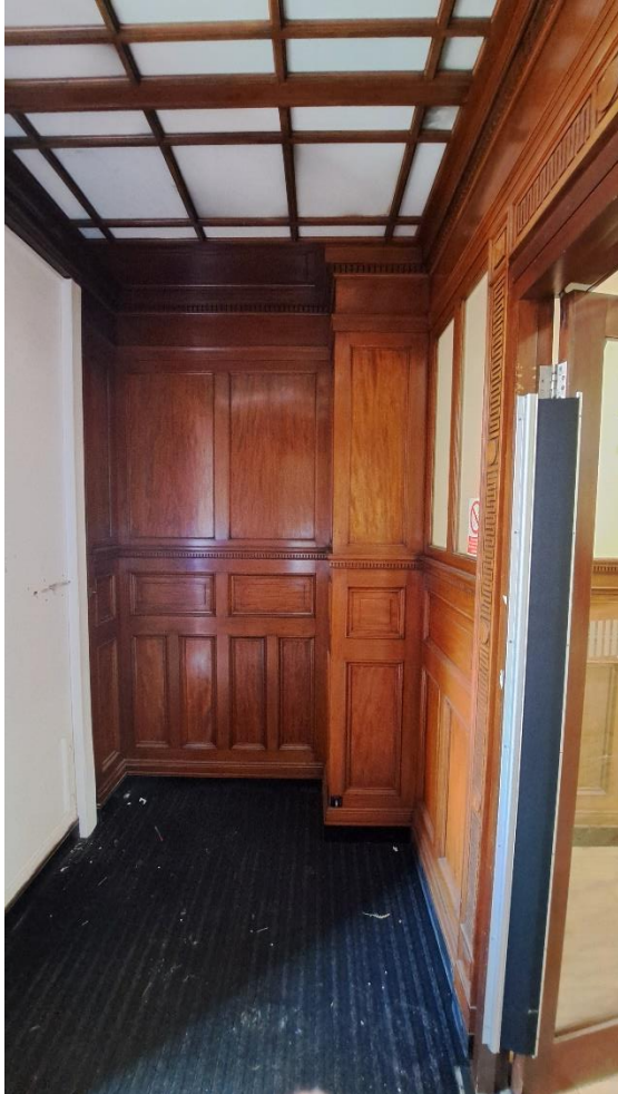
Figure 1 Vestibule with panelling and architraves
