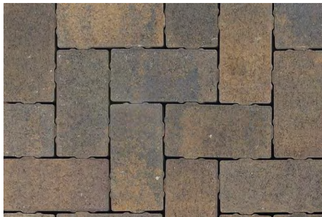
Car park permeable block paving (standard and accessible bays)
