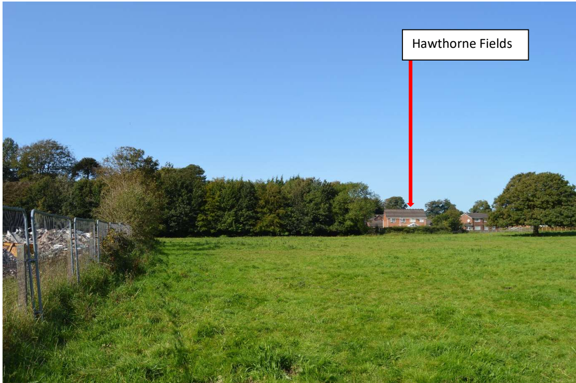
1a View north-westwards from the factory access road at the site boundary showing the mature trees which screens the Ennerdale Country House Hotel. The houses at Hawthorne Fields overlook the site.
