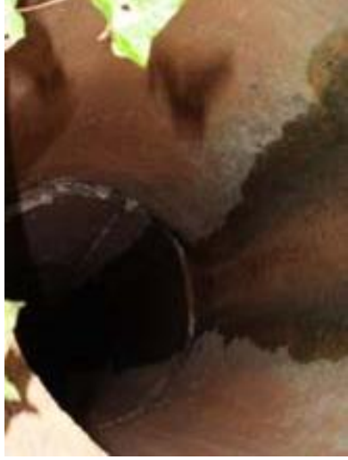
D/S 18" clay pipe flowing clear #1
