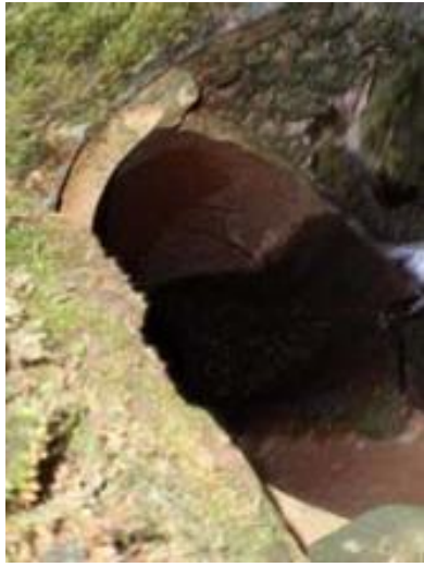
U/S broken 18" clay pipe
