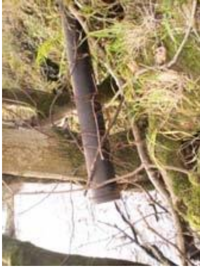
U/S broken 18" clay pipe
