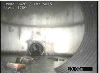
Settled deposits coarse 20% cross-sectional area loss - Remark: DEBRIS IN MANHOLE.
