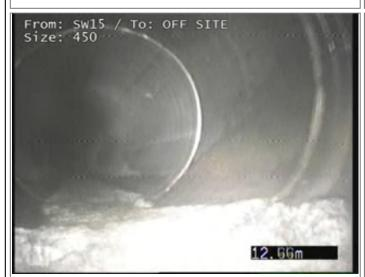
Joint displaced 10mm
