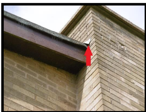
Plate 3: Lifted lead flashing.
