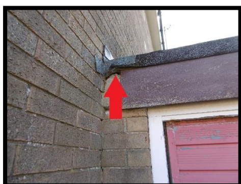
Plate 10: Missing mortar.
