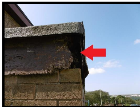
Plate 9: Gap in fascia board.
