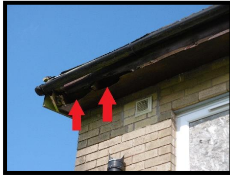
Plate 5: Gaps in soffit box.
