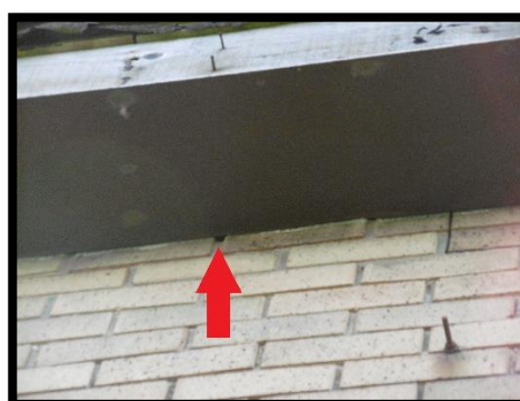
Plate 11: Gap at wallhead.
