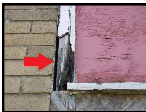
Plate 4: Gap in door frame.
