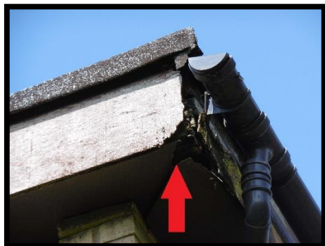
Plate 8: Gap in soffit box.
