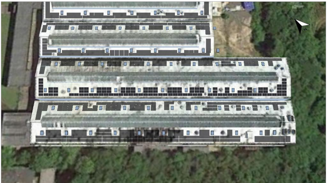
Figure: 5. Module Area - Building 02-Roof Area Southwest
