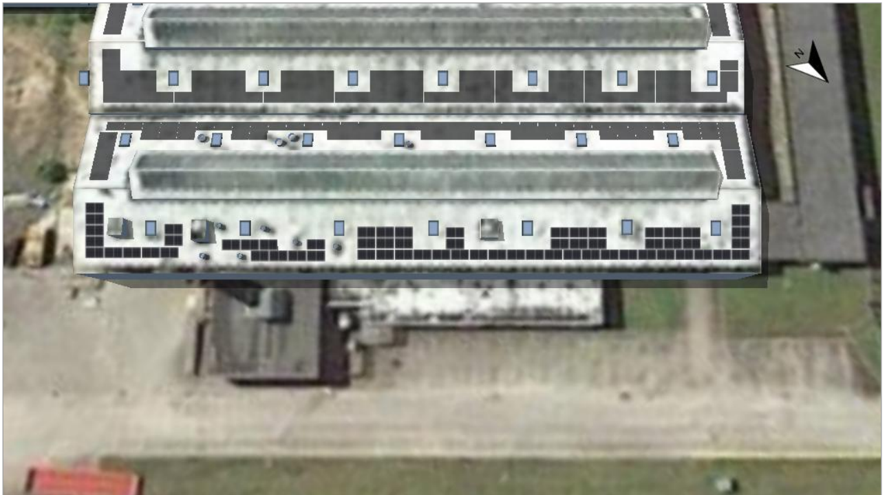
Figure: 4. Module Area - Building 04-Roof Area Northeast
