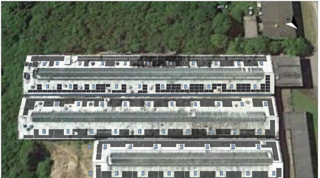
Figure: 2. Module Area - Building 01-Roof Area Northeast
