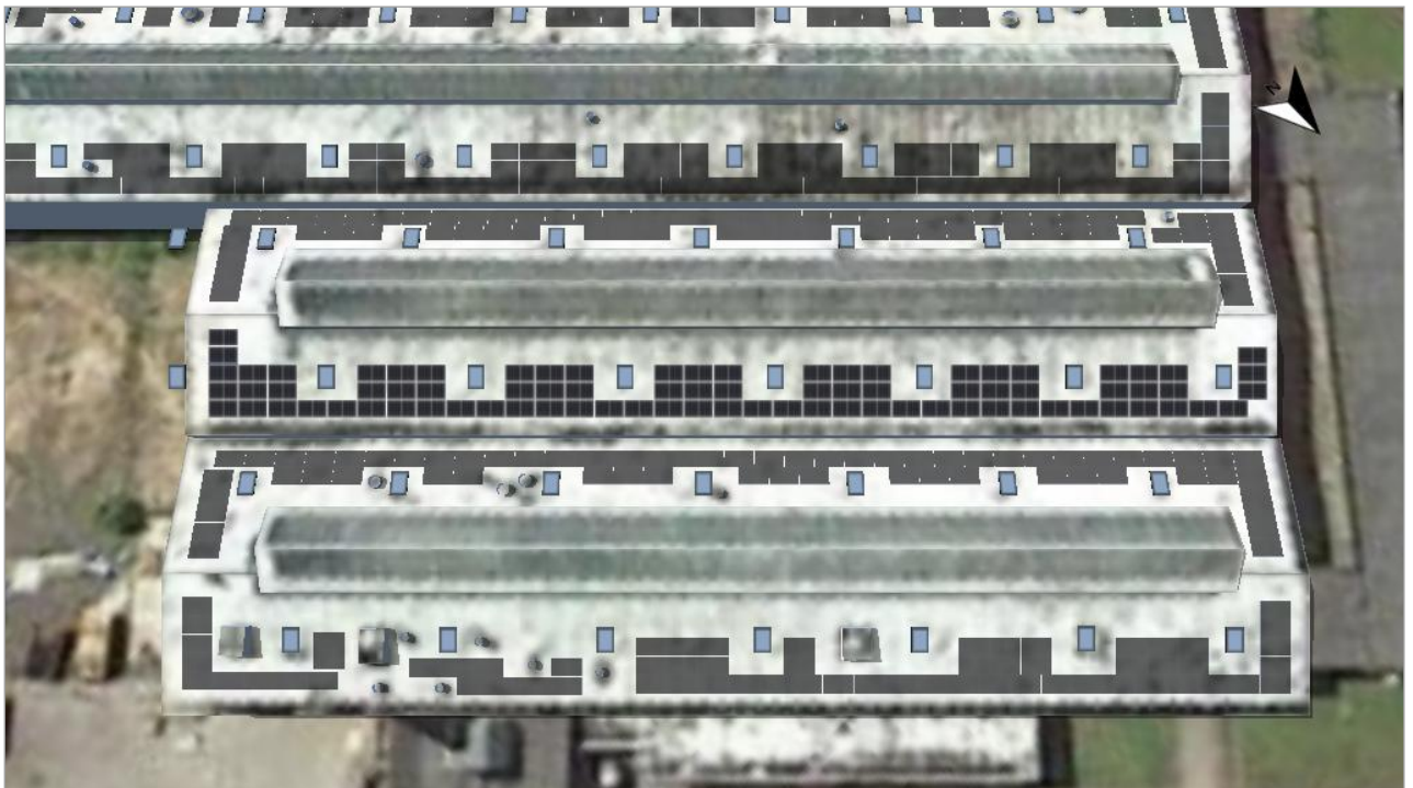
Figure: 8. Module Area - Building 03-Roof Area Northeast
