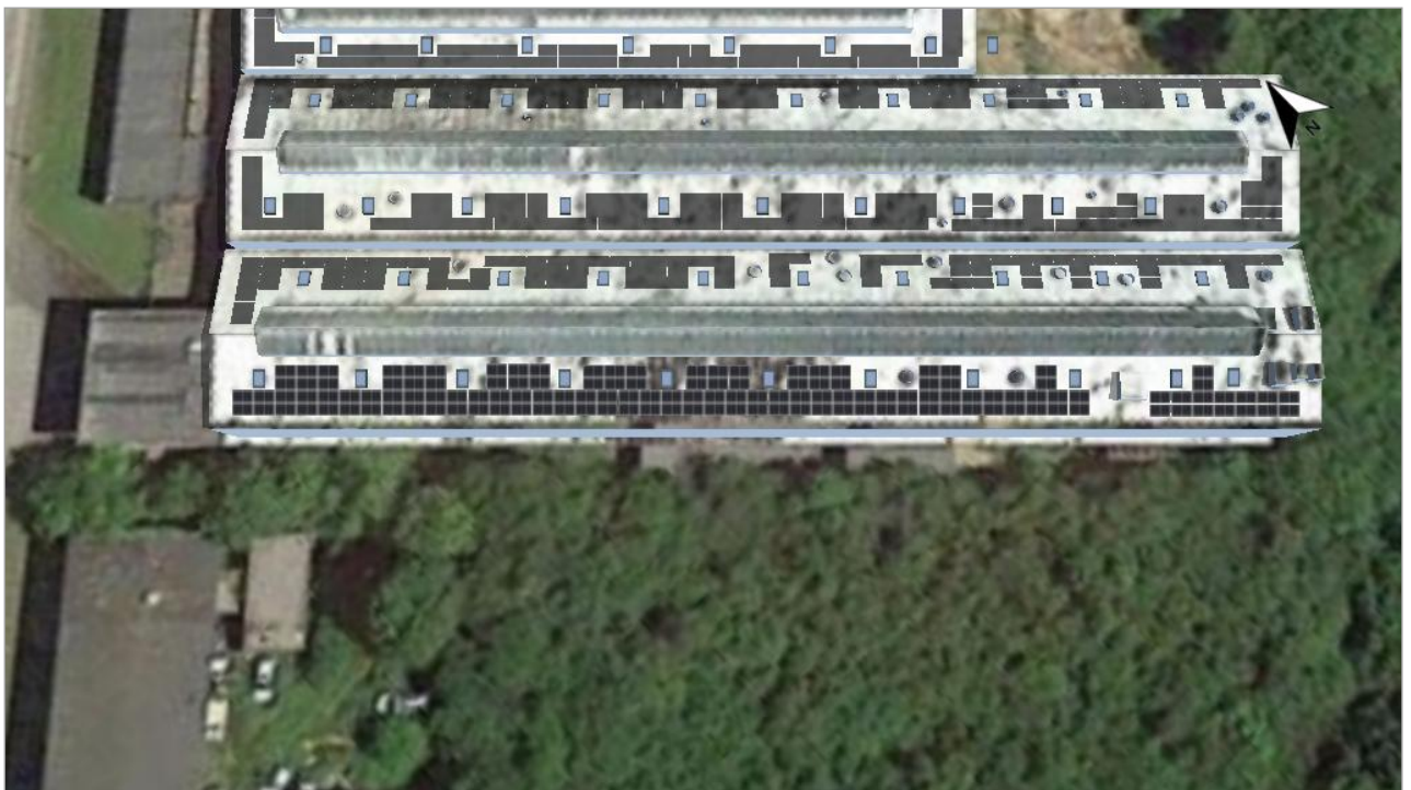
Figure: 1. Module Area - Building 01-Roof Area Southwest
