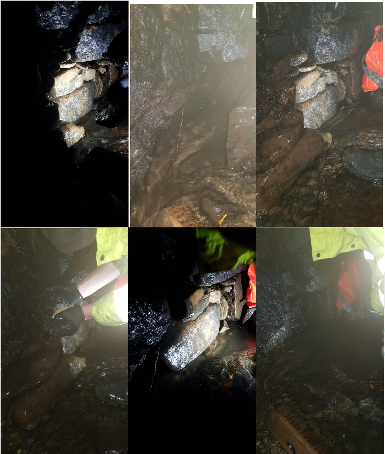
Stone retrieved from the culvert being used for repairing
