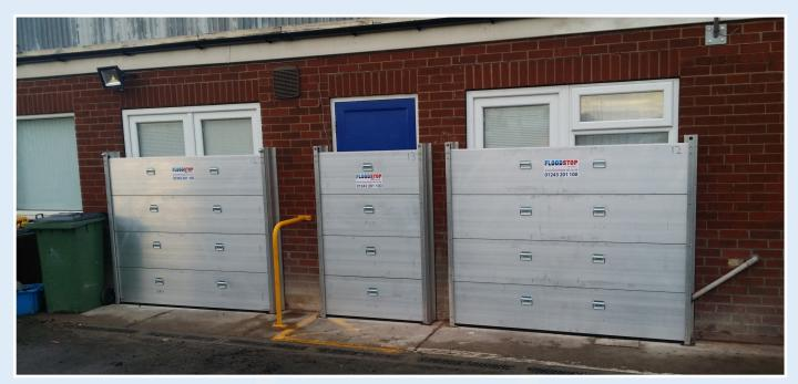
2000mm wide, 1125mm wide and 2100mm wide. All are at 1600mm high (4 panels). All are face fixed with 100mm deep packers to bring the flood barriers forward to clear the door cills and security entry pads.
