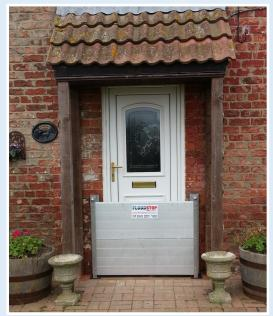
920mm wide x 800mm high (2 panels) with 75mm packers to bring the flood barrier forward to clear the door cill. Face fixed.
