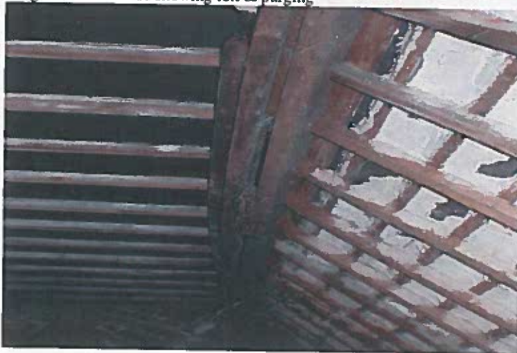
Ridge beam of house showing felt & parging
