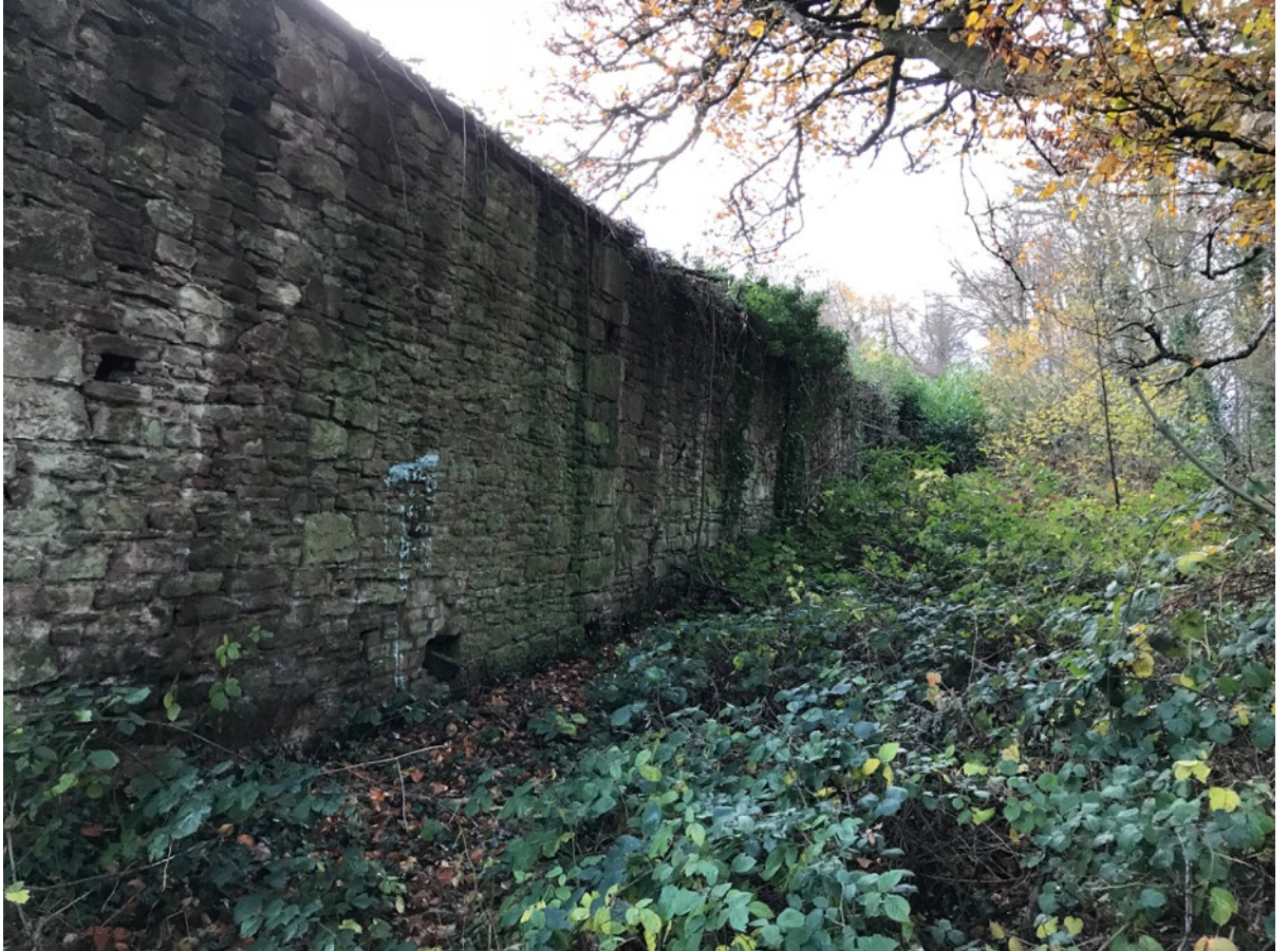
Photograph 9. Exterior of wall forming allotment perimeter
