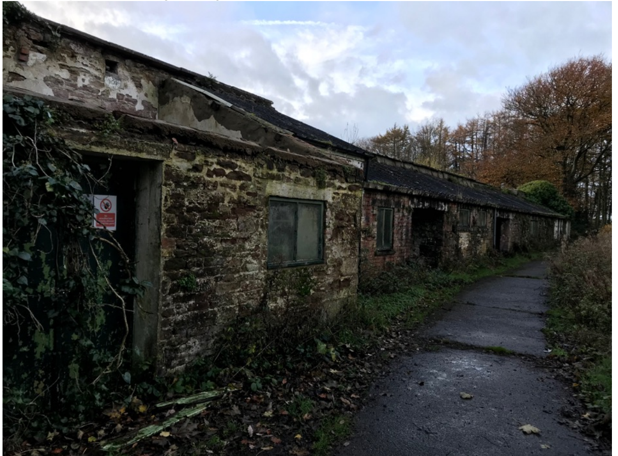
Photograph 2. Building 1, adjacent to northern wall
