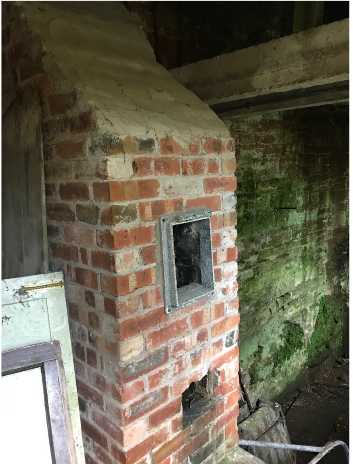
Photograph 3. Former boiler room, within Building 1
