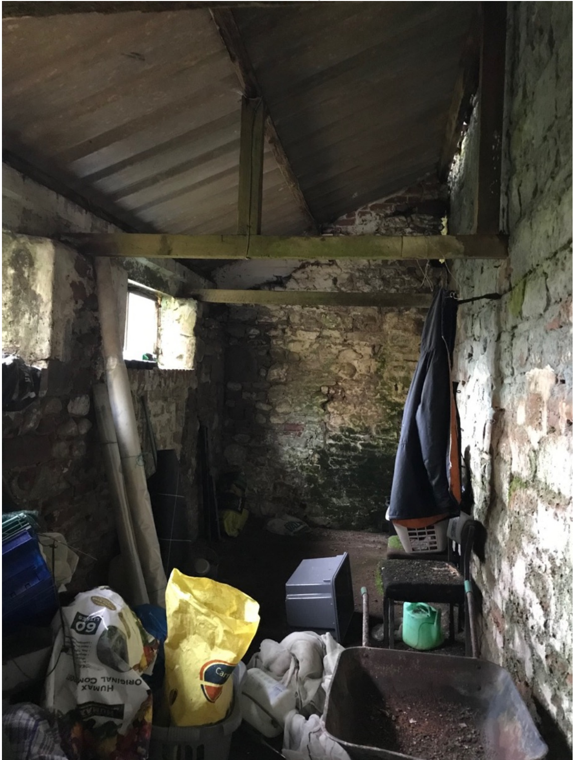
Photograph 4. Interior of a section of Building 1
