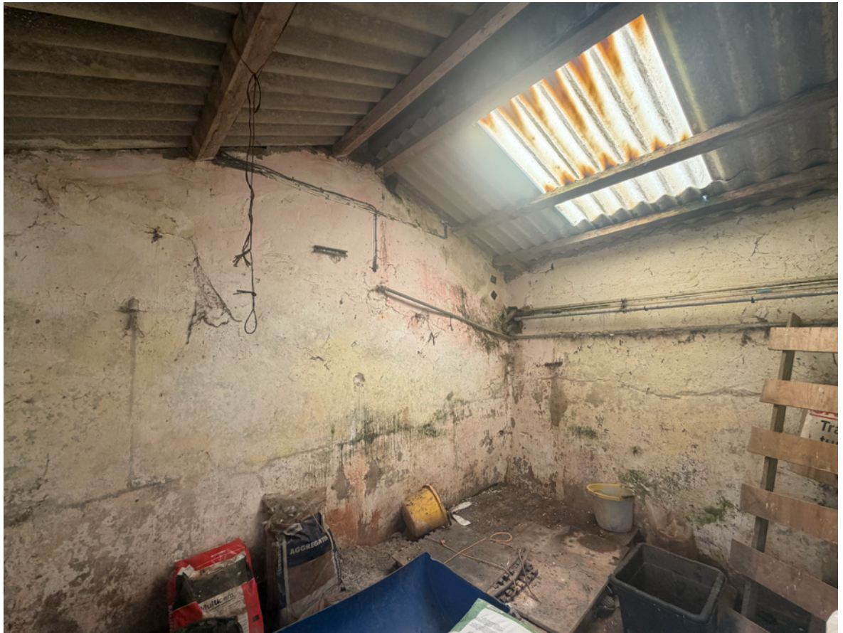
Photograph 2. Typical interior of building within the site (03/06/2026)
