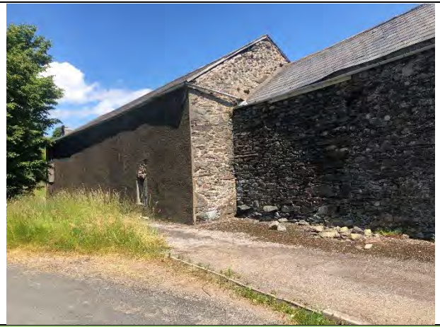
P2: A cluster of two attached farm buildings of stone construction with slate roofs are situated in the north-west of the site
