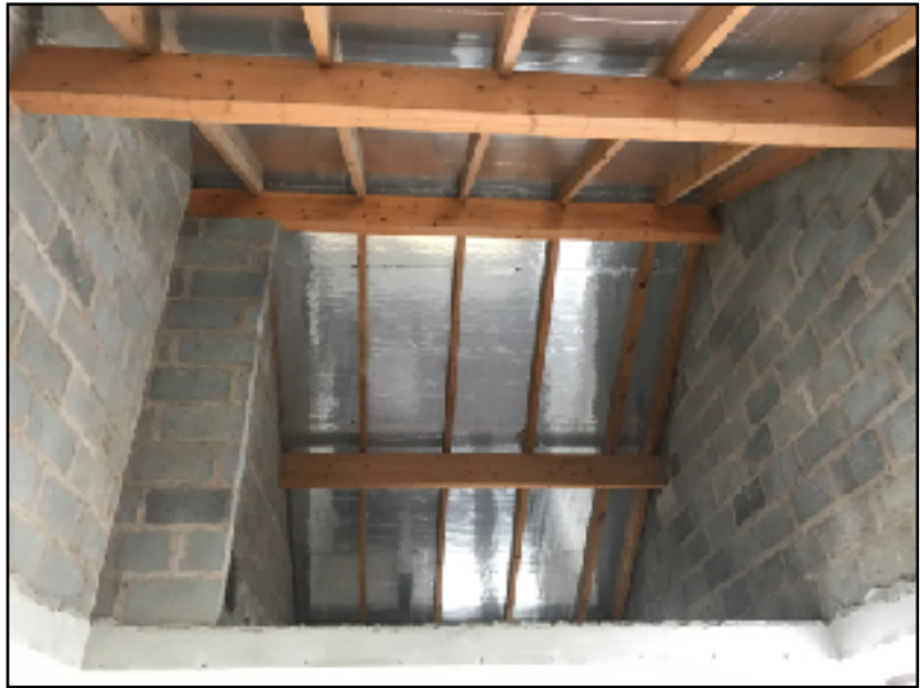
Figure 2: Showing example of the rigid panel insulation.
