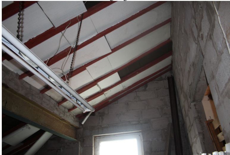
Internal view of west garage with insulation between rafters
